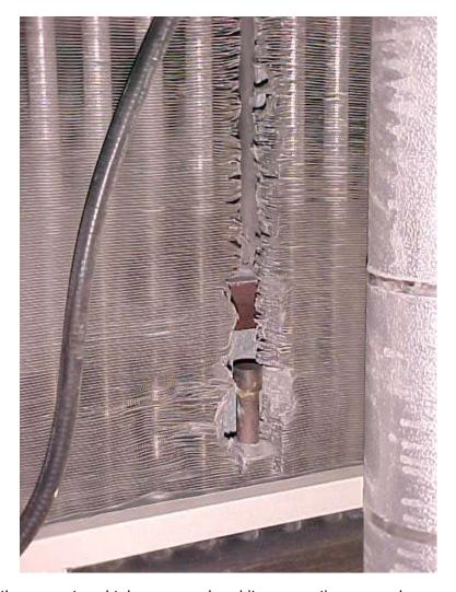
Steam coil with one ruptured tube removed and its connection capped
