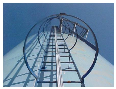
Photo # 4—STGTGS--- Fuel Storage Tank with T-Rail Attached to Ladder
