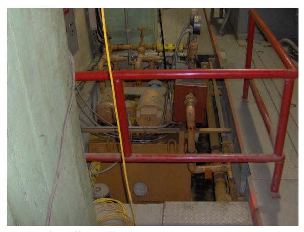
Figure 15- Main Lube Oil Pump (2005)
