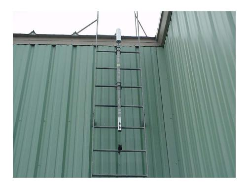
Photo # 2---Natuashish Diesel Plant---T-Rail attached to Building Access Ladder.
