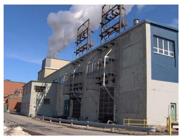
Figure 13 – Towers and External 66 kV Bus (2005)
