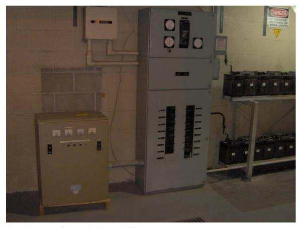
Figure 9 – Battery Charger & DC Panel (2005)
