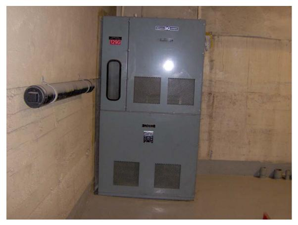
Figure 7 – Neutral Grounding Transformer (2005)
