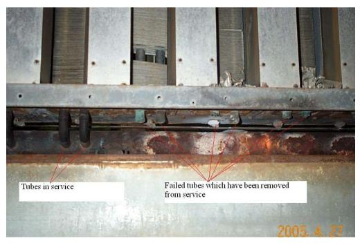
Steam coil section with failed tubes
