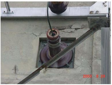
Damaged A phase entrance insulator.
