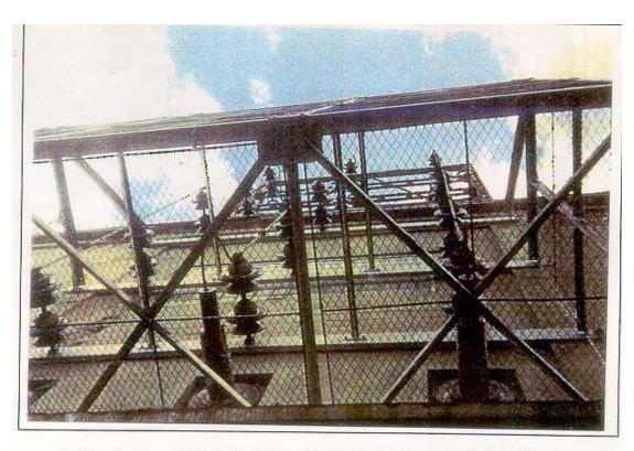
Photo 3: Damaged bushings outside the converter building - August 19, 1998
