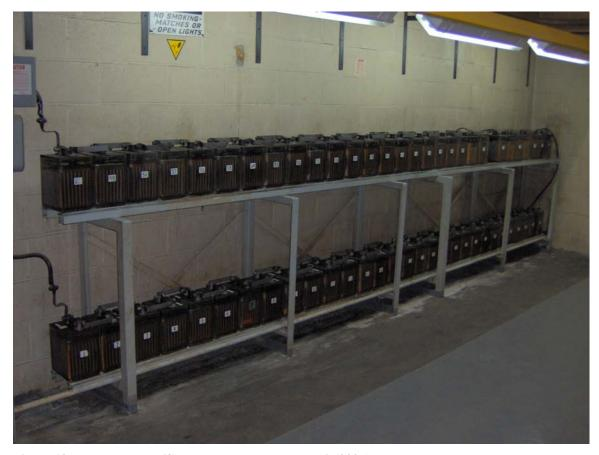
Figure 10 – Battery Bank (Scheduled For Replacement) (2005)
