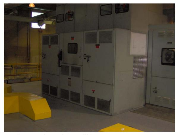
Figure 16 – Frequency Converter Switchgear (2005)
