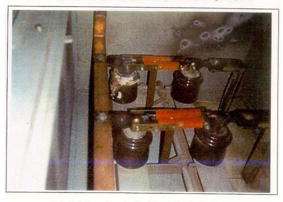
Photo 2: Arcing and burning found in cubicle - August 19, 1998
