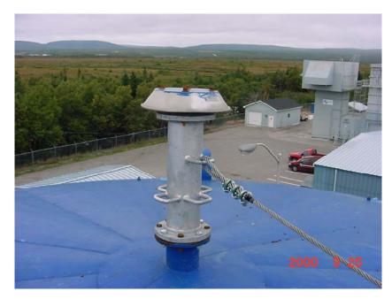
Photo # 5—STGTGS Fuel Storage Tank with Safety Wire Attached to Tank Center Vent
