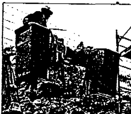
Above: Lineman Lonz Pearce removes reusable pieces from a utility pole that fell under the weight of wet snow and ice in this week's storm. Below left: Lineman Todd Noseworthy installs the cross brace on a new telephone pole near the Coast Guard building on the southside of St. John's. The pole it replaces broke under the weight of snow. Below right: Lineman Ian Costello has been climbing utility poles for 25 years.
