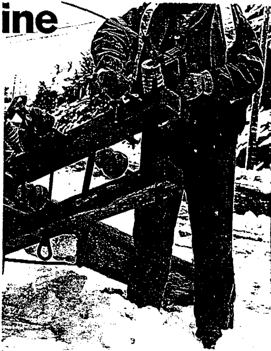
Above: Lineman Lonz Pearce removes reusable pieces from a utility pole that fell under the weight of wet snow and ice in this week's storm. Below left: Lineman Todd Noseworthy installs the cross brace on a new telephone pole near the Coast Guard building on the southside of St. John's. The pole it replaces broke under the weight of snow. Below right: Lineman Ian Costello has been climbing utility poles for 25 years.
