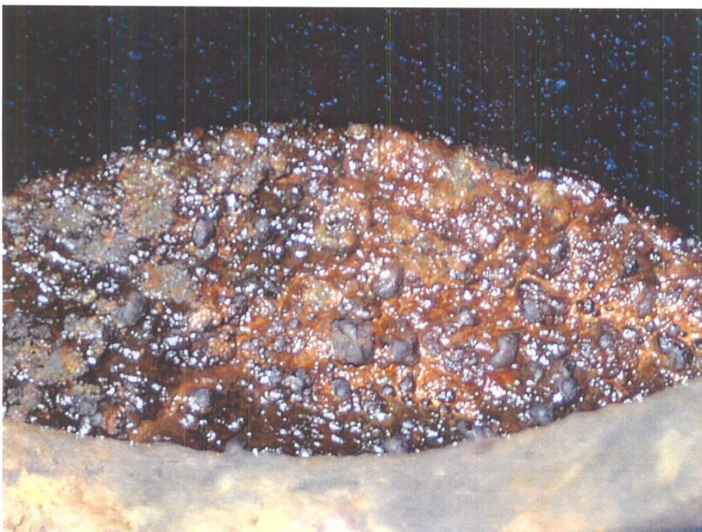
Growth on Internal Surface of Penstock
