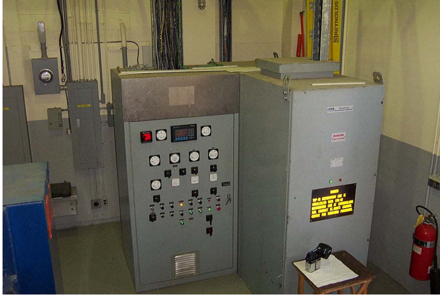
Unit Control Panel and Generator Breaker
