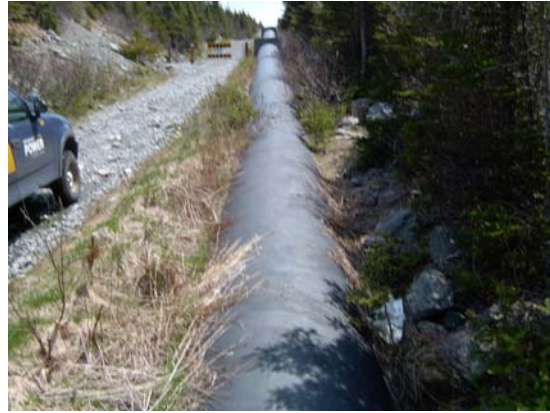
Section of Steel Penstock Half Buried
