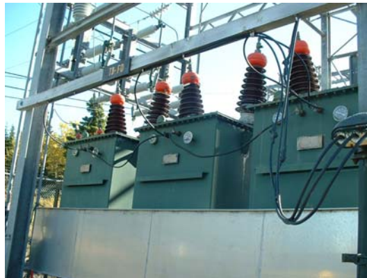
Station Service Transformers
