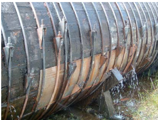
Steel Plate Bridging Missing Woodstave
