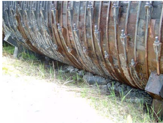
Penstock in Contact with Ground
