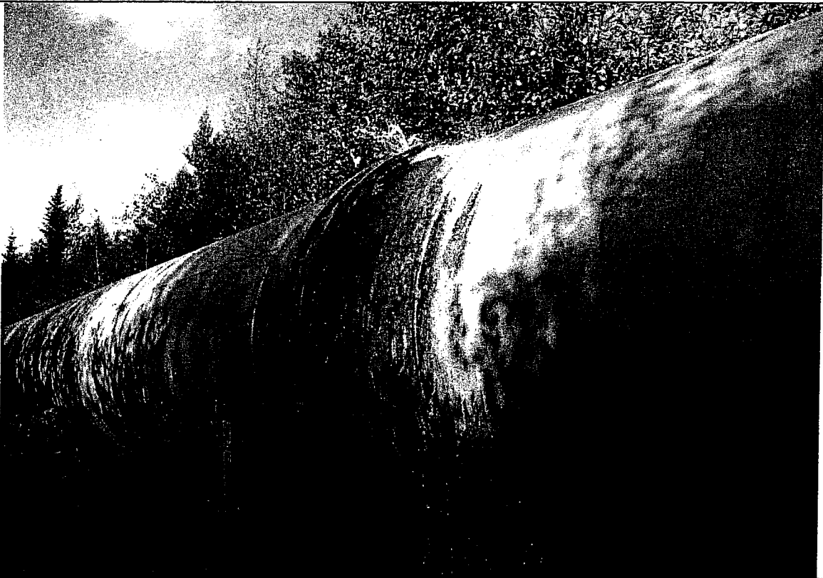
12. Expansion joint #2 leaking at top.
