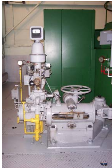
Unit #1 Governor Control And Wicket Gate Actuator
