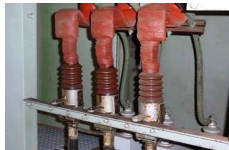
Unit #1 Generator Cable Terminations
