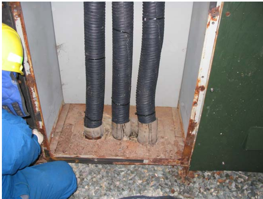
St. John's Main Substation Deteriorated Metal Clad Switchgear Picture #1
