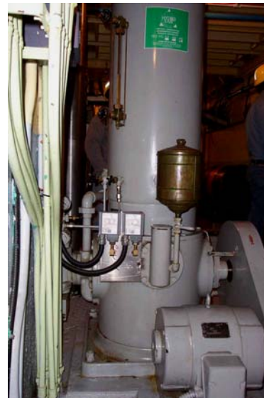
Unit #1 Oil Accumulator And Governor Oil Pump
