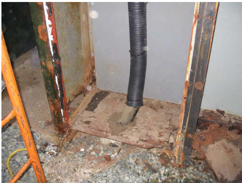
St. John's Main Substation Deteriorated Metal Clad Switchgear Picture #3
