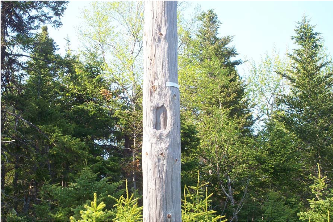
Figure 4 Deteriorated pole 110L
