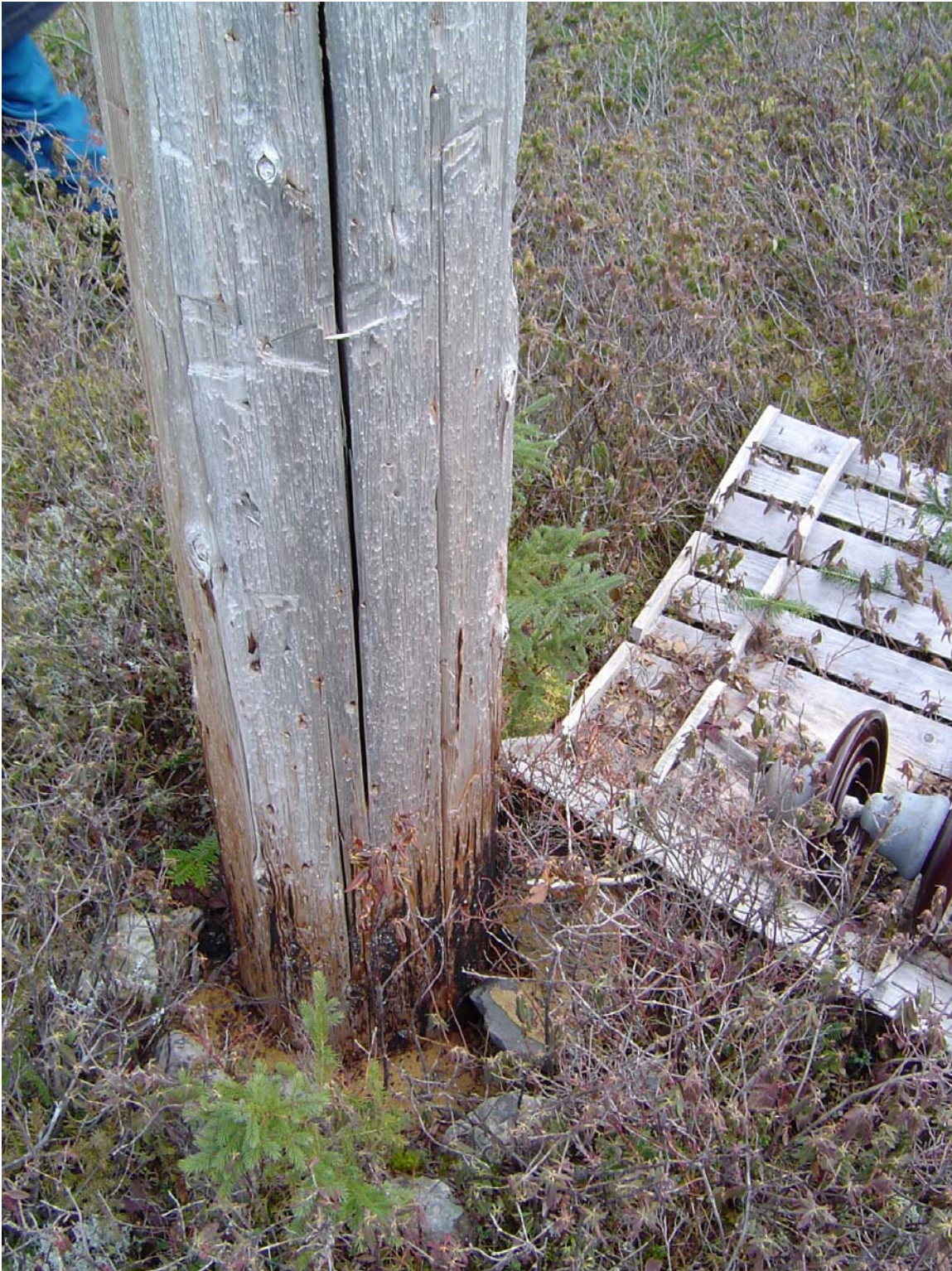
Figure 6 Deteriorated pole (ant damage) 43L
