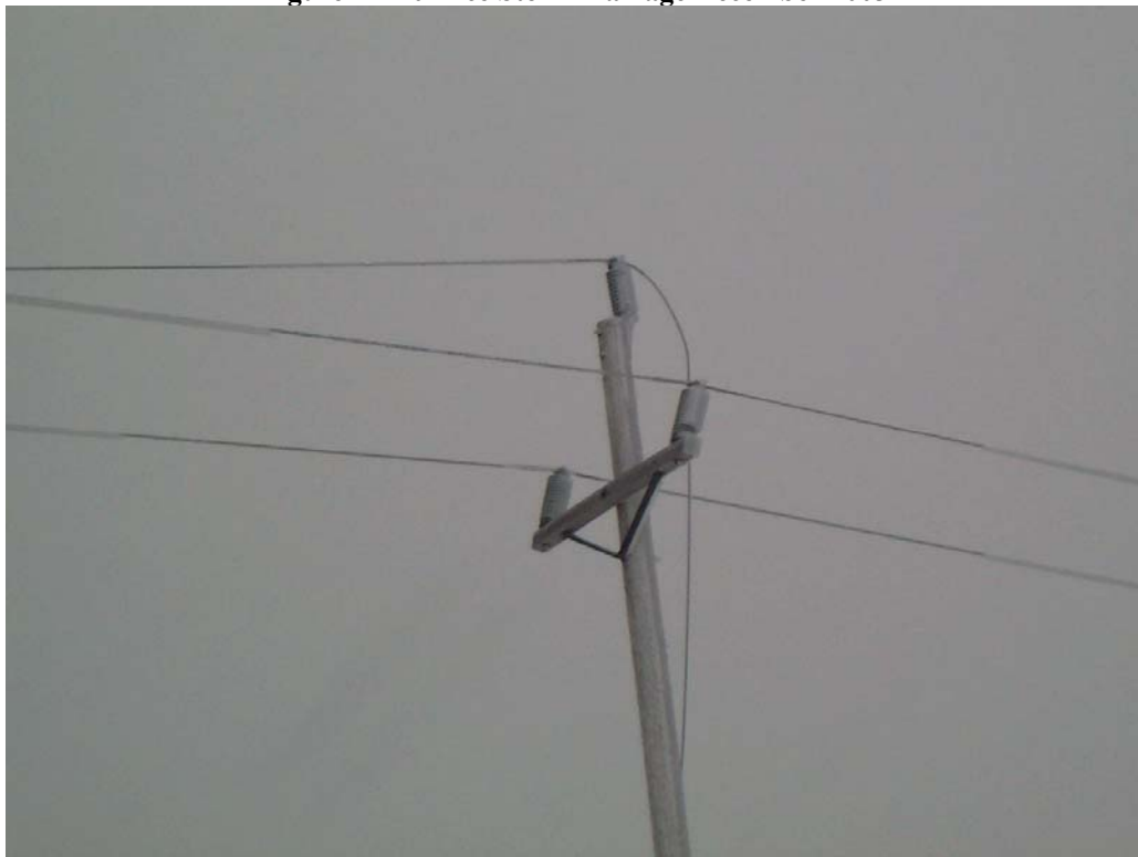
Figure 3 110L Broken conductor - ice build up December, 2003
