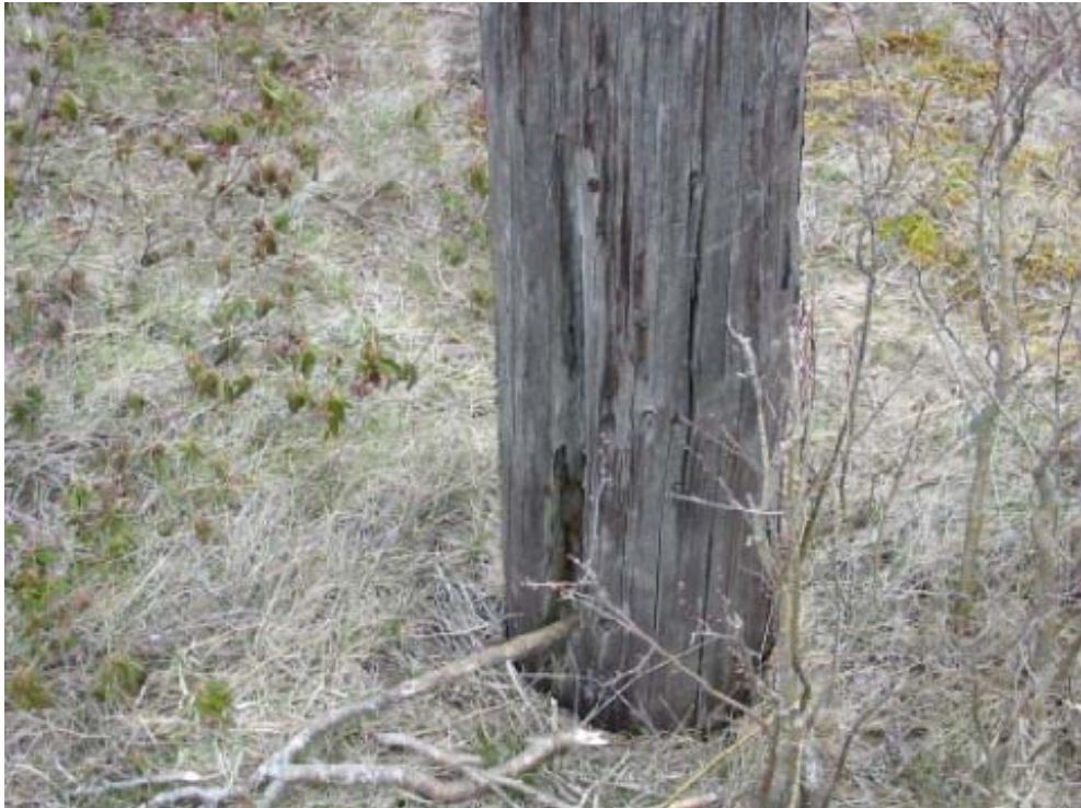
Figure 2 Deteriorated pole 407L
