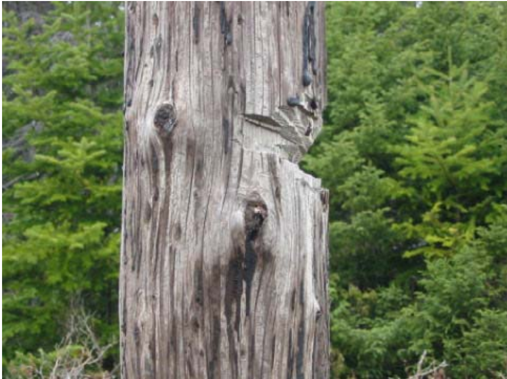
Figure 4 Vandalized pole 407L
