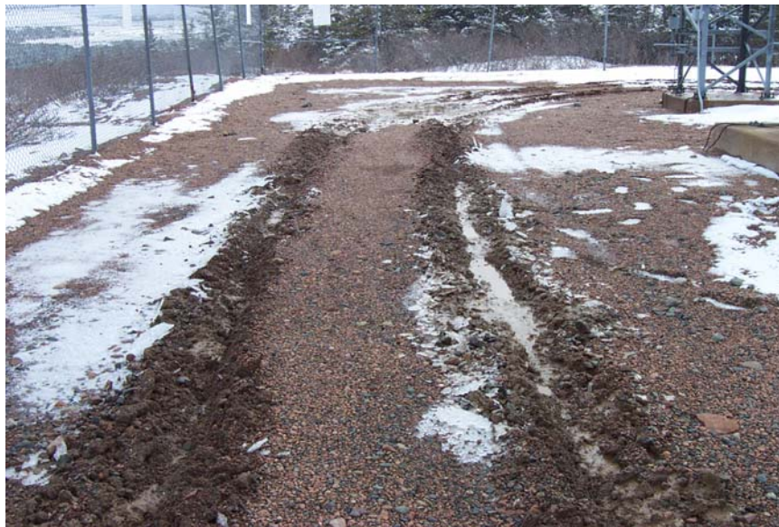
Picture #2: Laurentian Substation Damage to crushed stone and sub-grade.
