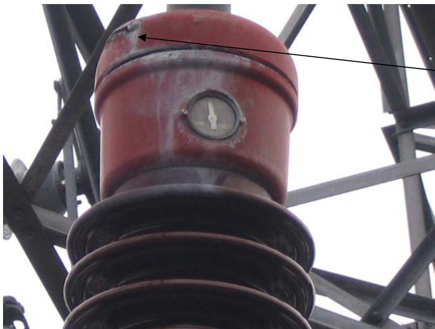
Picture 2 Bushing Deterioration
