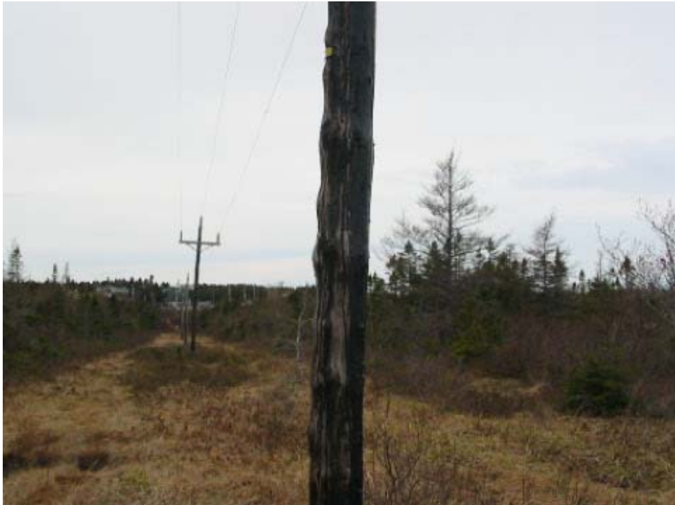
Figure 6 Deteriorated pole 407L
