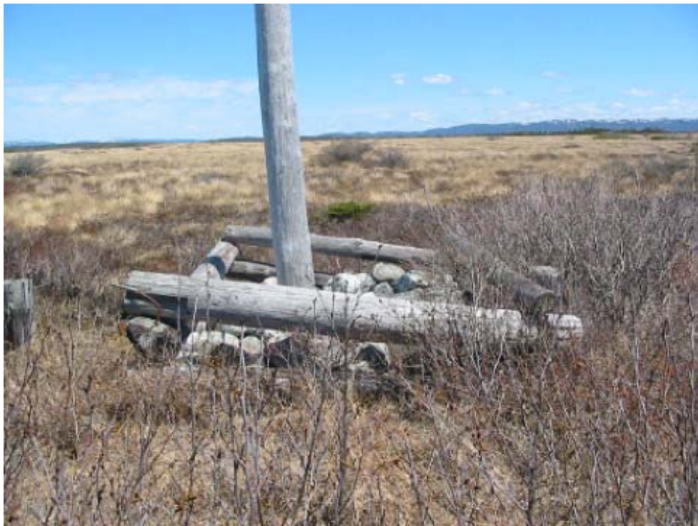
Figure 3 Deteriorated crib 407L
