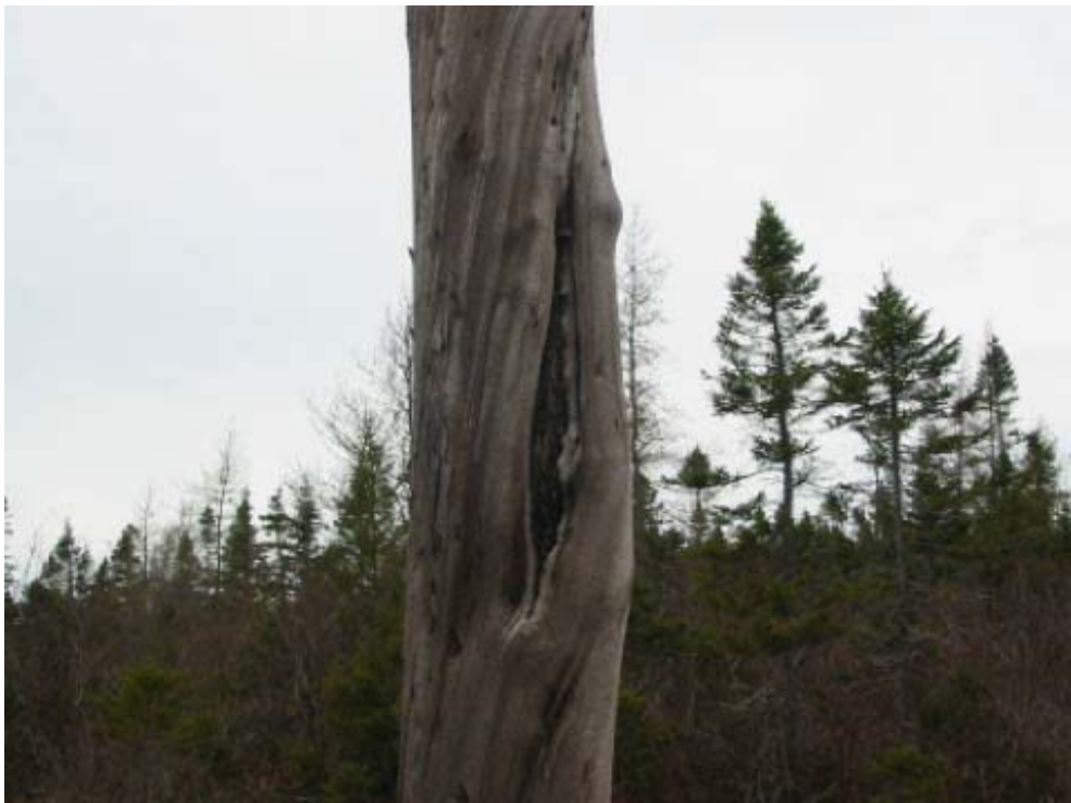
Figure 7 Deteriorated pole 407L
