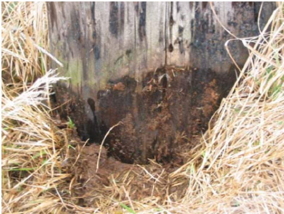
Figure 5 Ground line decay 407L
