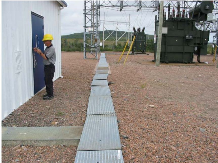
Picture #1: Laurentian Substation Shifting of cable trench due to frost heaving.
