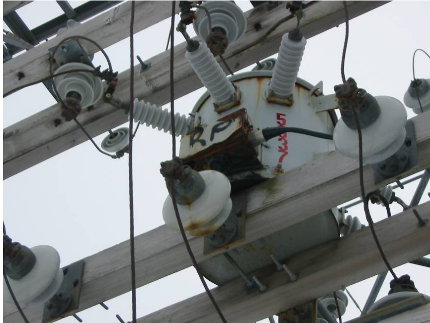
Corrosion damage Garnish Substation
