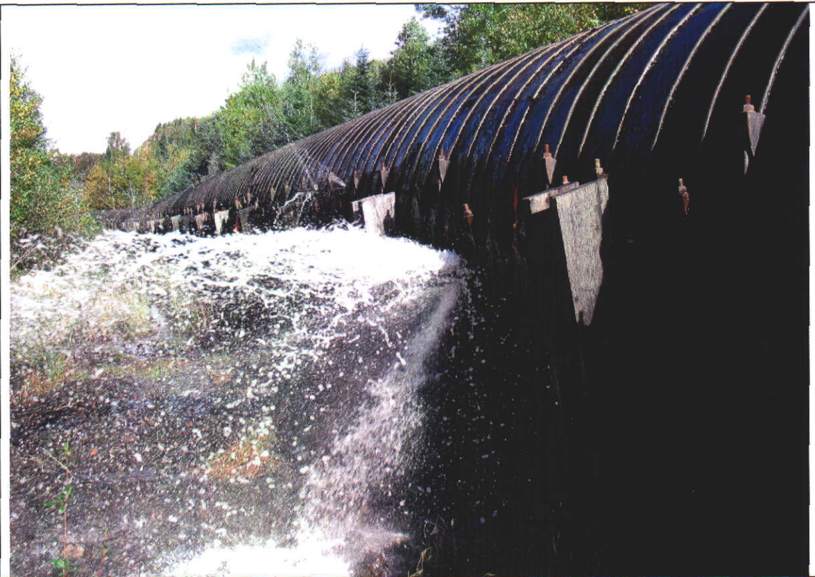
17. Wood stave penstock leakage.
