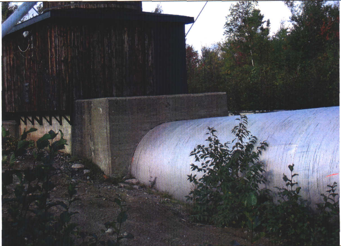
13. Surge tank anchor block with shrinkage crack.
