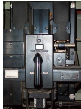
Figure 6 - Field Breaker
