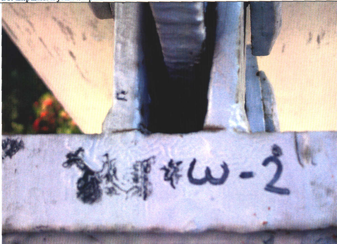
22. Horizontal brace north face at leg #3. Cracks in welds.
