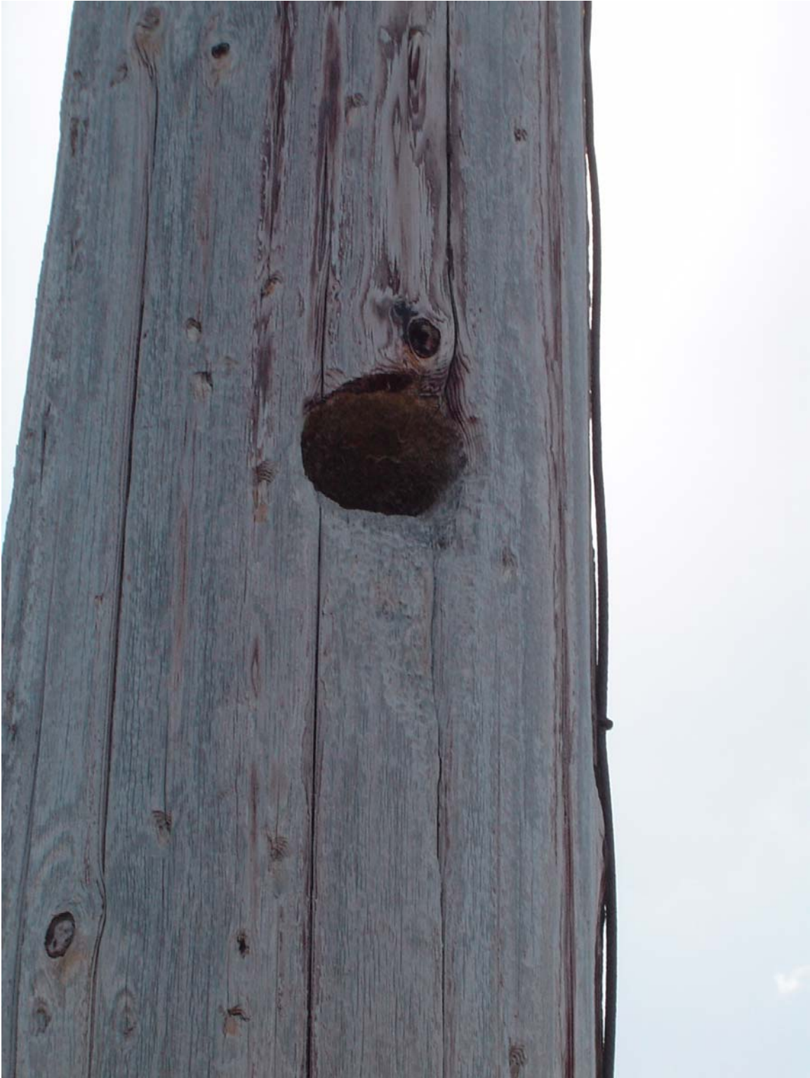
Figure 4 - Woodpecker damage 43L
