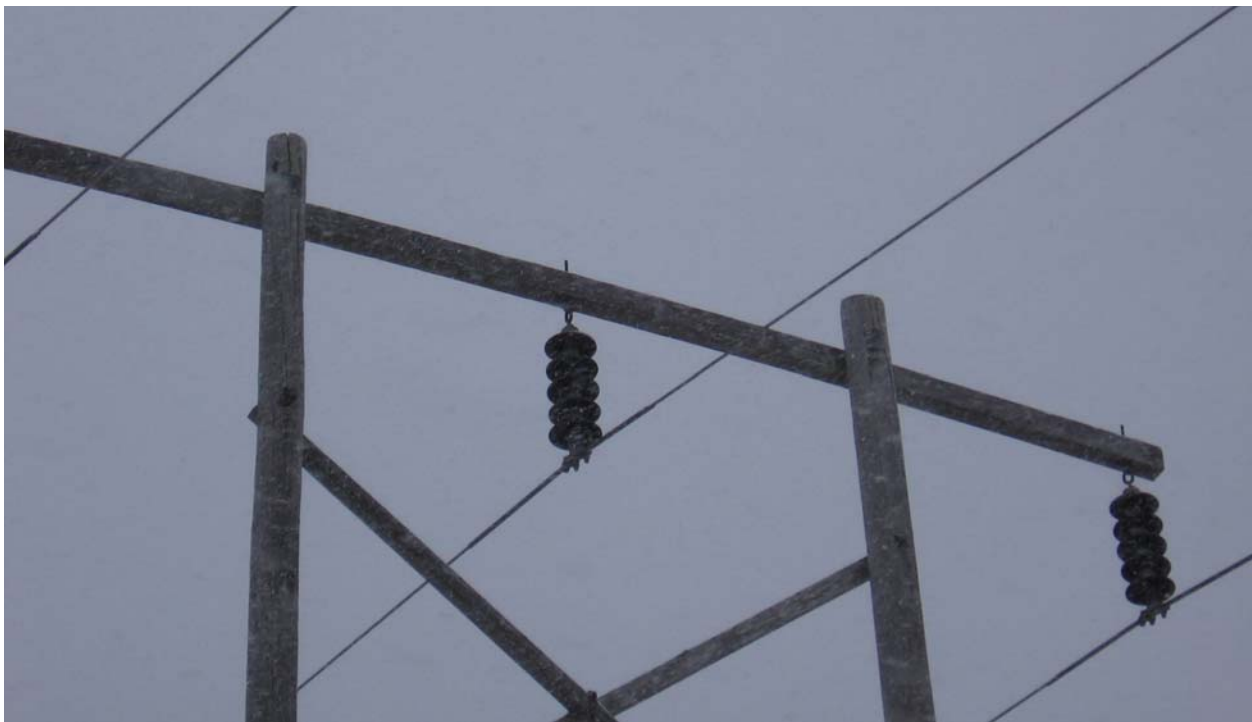
Figure 13 - Deteriorated Poles (top split) 20L
