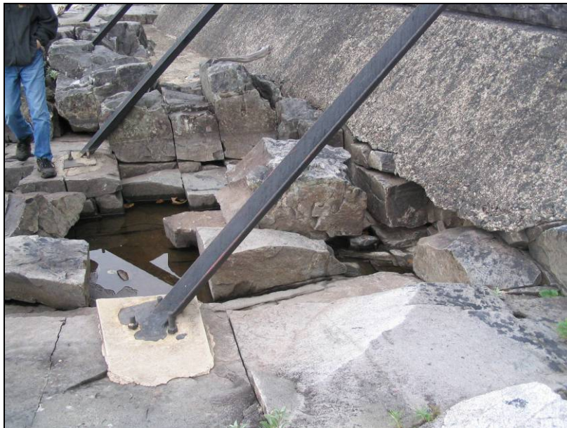
Figure 2: Undercutting of Concrete/Bedrock Interface
