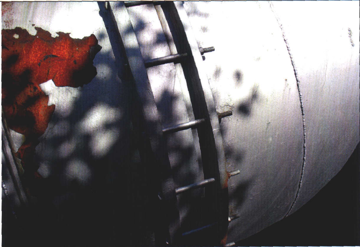
21. Expansion joint #1 paint failure.
