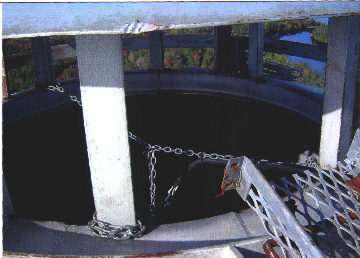
1. Rolling platform loose expanded metal mesh.
