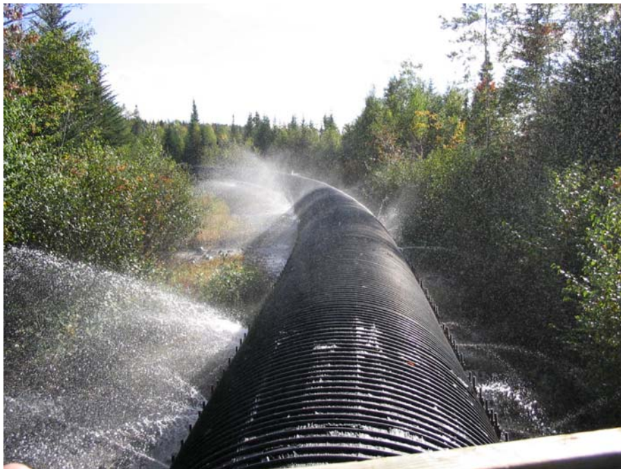
Figure 4: Water Leakage from Penstock
