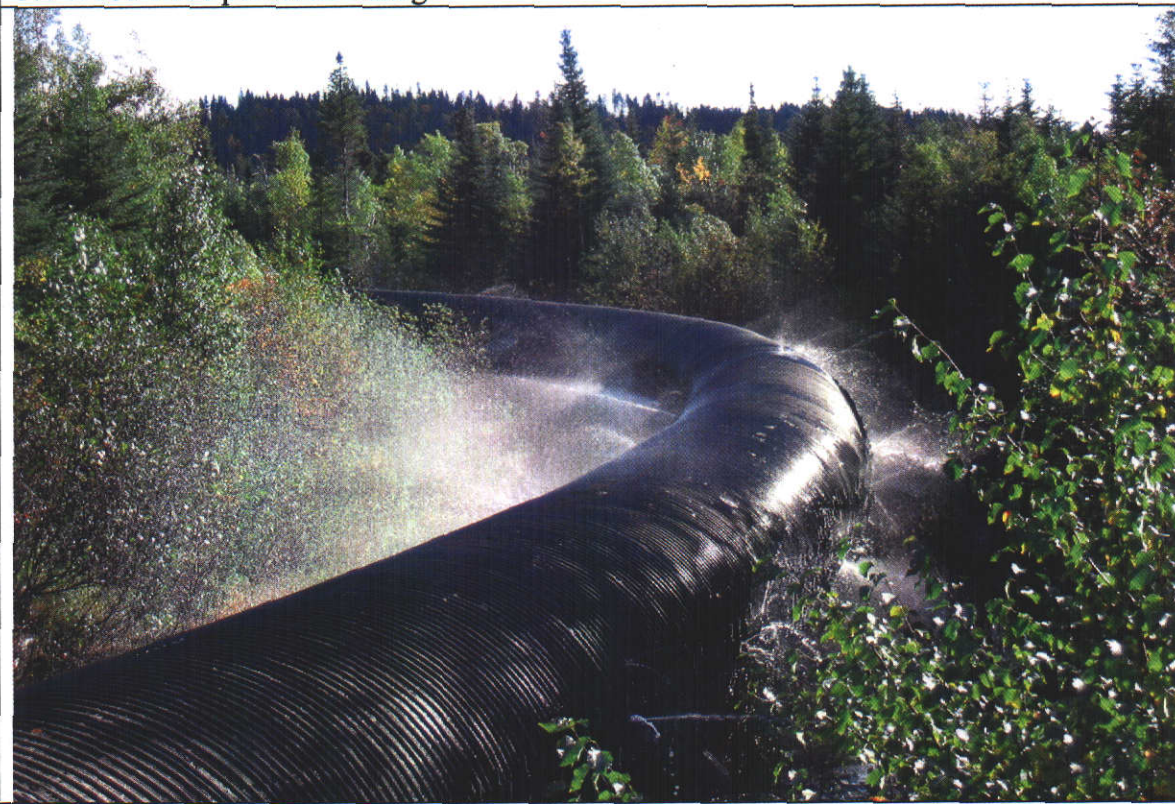
18. Wood stave penstock leakage.
