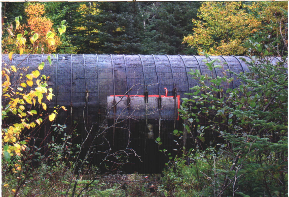
14. Wood stave penstock steel plate patch.
