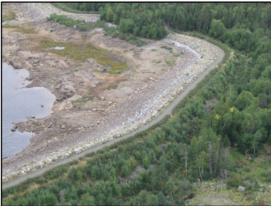
Figure 4: Rattling Lake Dam (Note excessive vegetation on downstream face)
