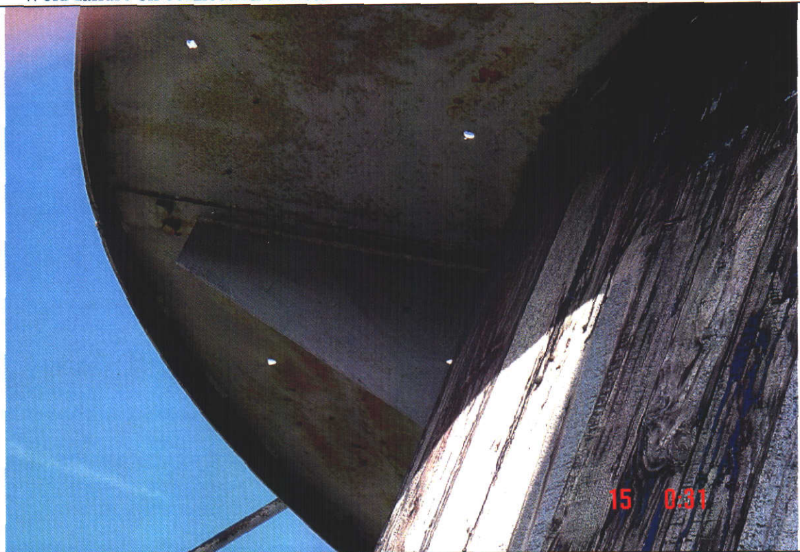
6. Compression ring and walkway at EL.207'.
