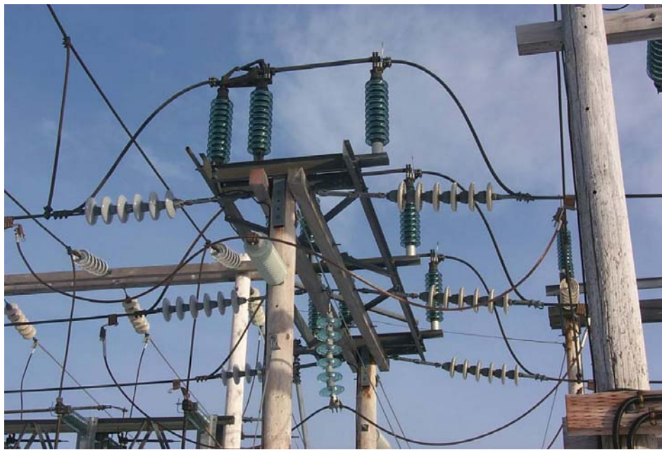
Bus Tie Switch Bypassed Goulds Substation
