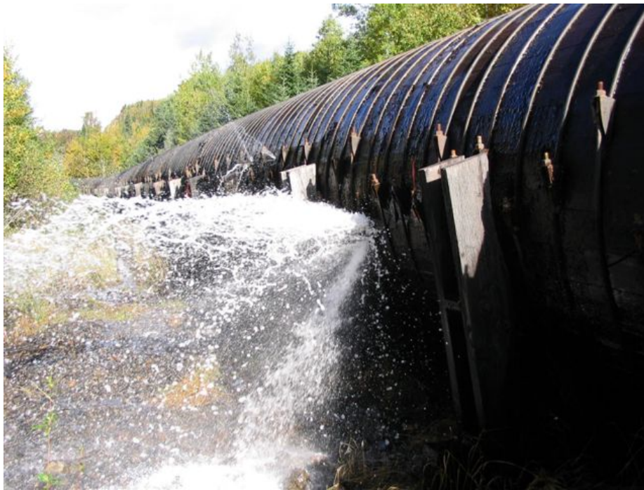
Figure 1: Water Leakage from Penstock
