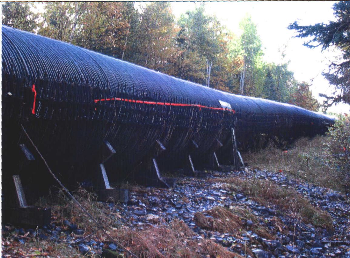
15. Wood stave penstock typical patch plate location marking.
