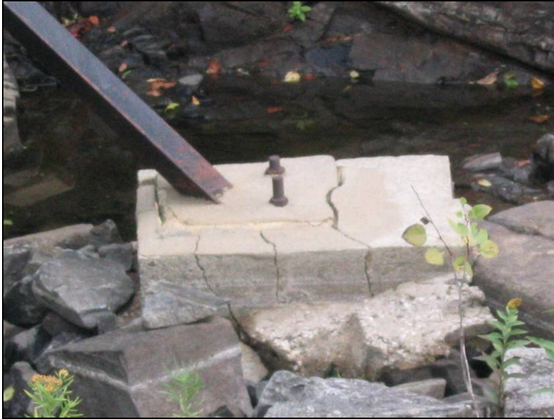
Figure 3: Fractured Brace Foundation
