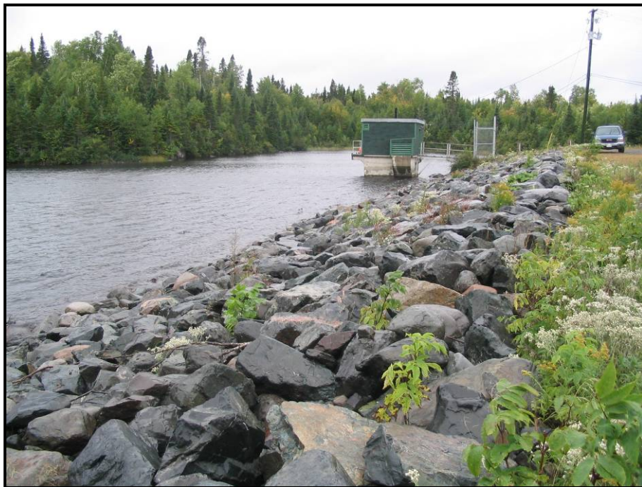
Figure 12: Forebay Dam (Upstream Face)
