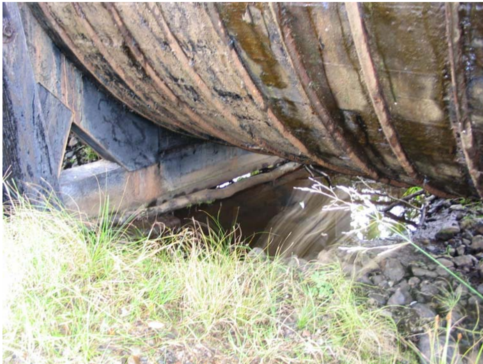
Figure 13: Undermining of Penstock Bedding
