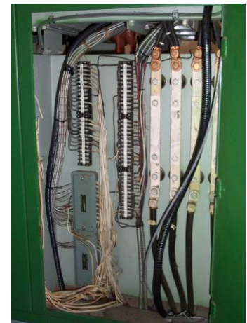
Figure 4 – Termination Cabinet
