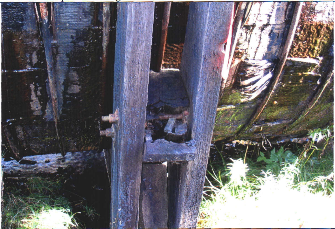
20. Wood stave penstock saddle deterioration.
