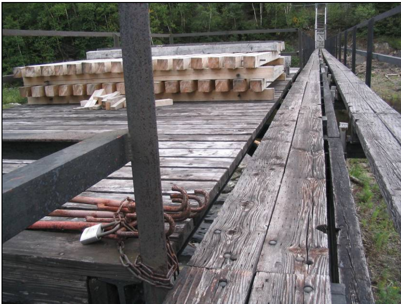
Figure 4: Deteriorated Walkway Timbers & Operation Staff's "Removal" System
