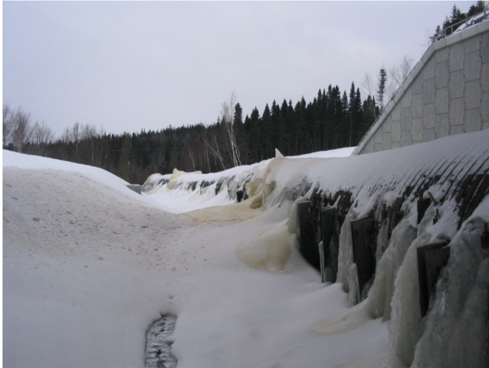
Figure 10: Ice Forming on Penstock during Winter
