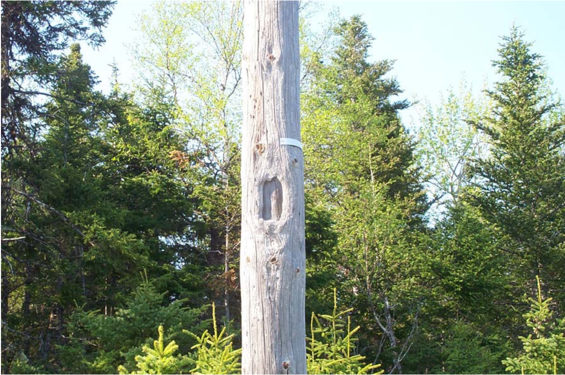
Figure 8 - Deteriorated pole 110L
