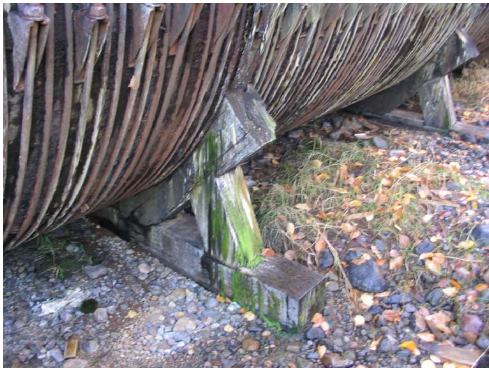
Figure 11: Settlement of Penstock Supports
