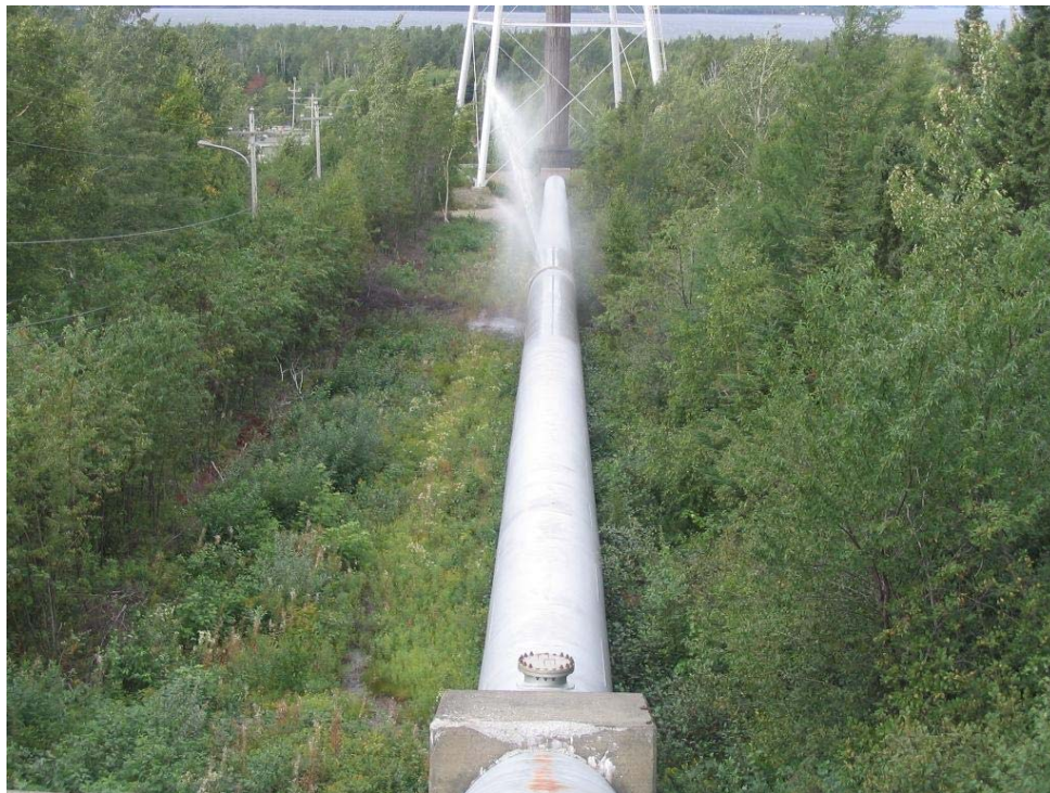
Figure 19: Leakage at Expansion Joint
