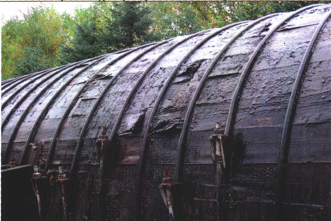
16. Wood stave penstock surface condition.
