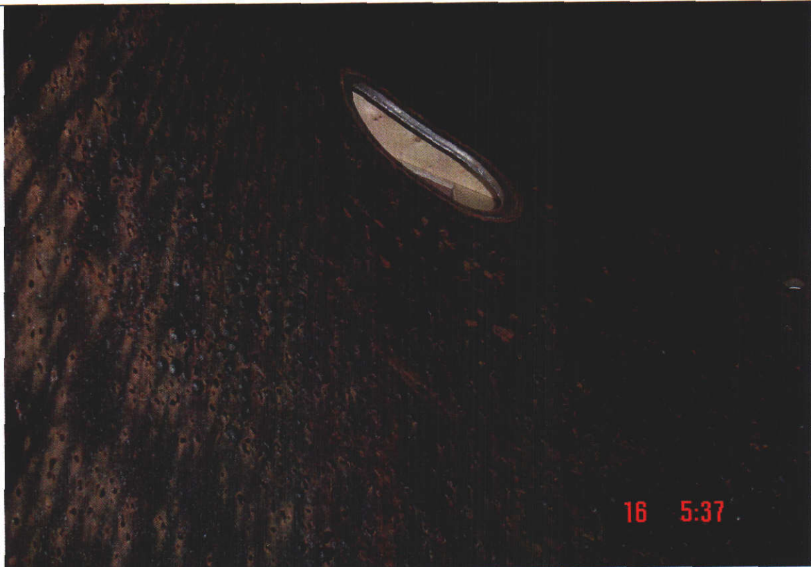
9. Surface corrosion of surge tank tee at access hatch.
