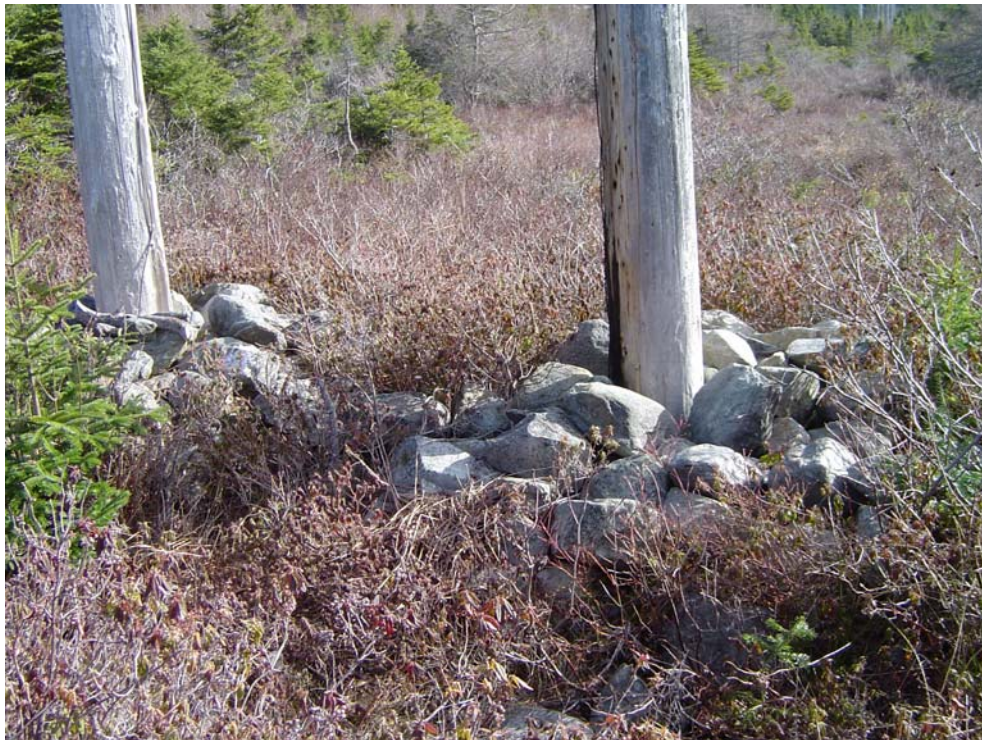
Figure 3 - Deteriorated cribs 43L
