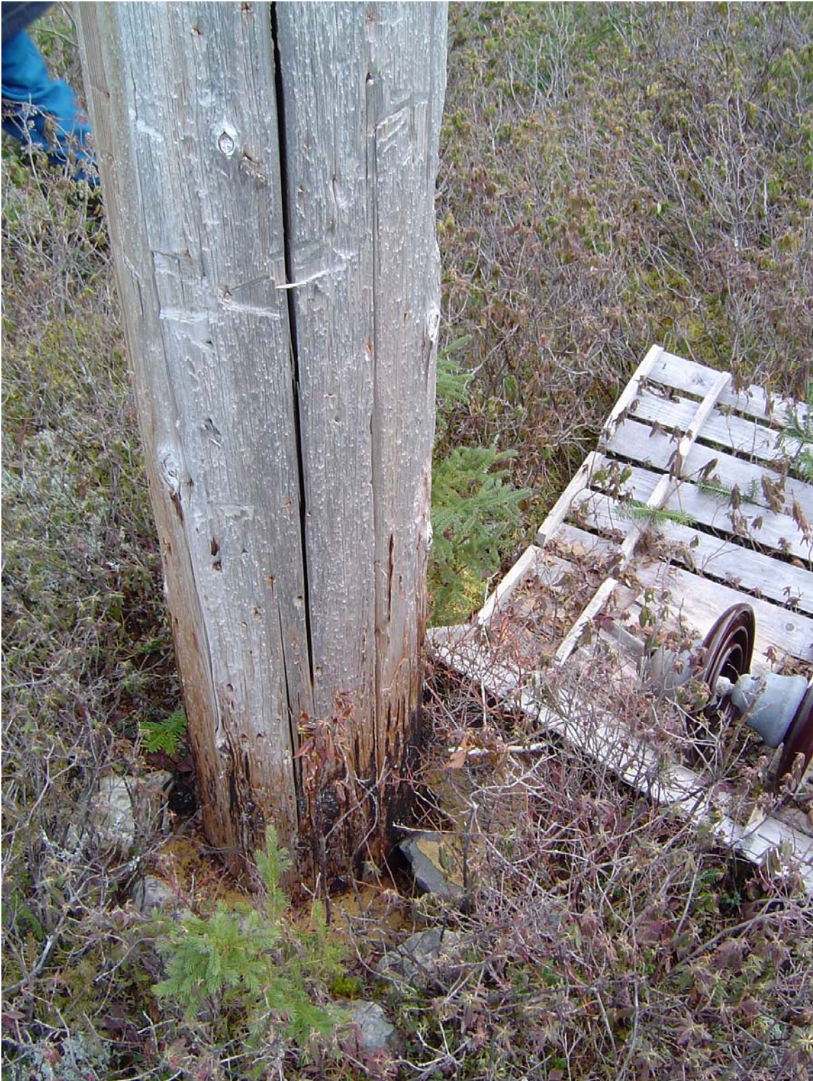
Figure 5 - Deteriorated pole (ant damage) 43L
