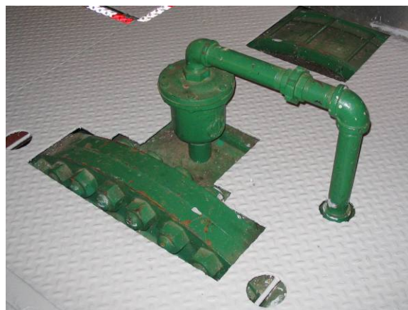
Figure 10 – Scroll Case Air Vent
