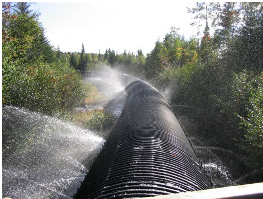
Figure 2: Water Leakage from Penstock
