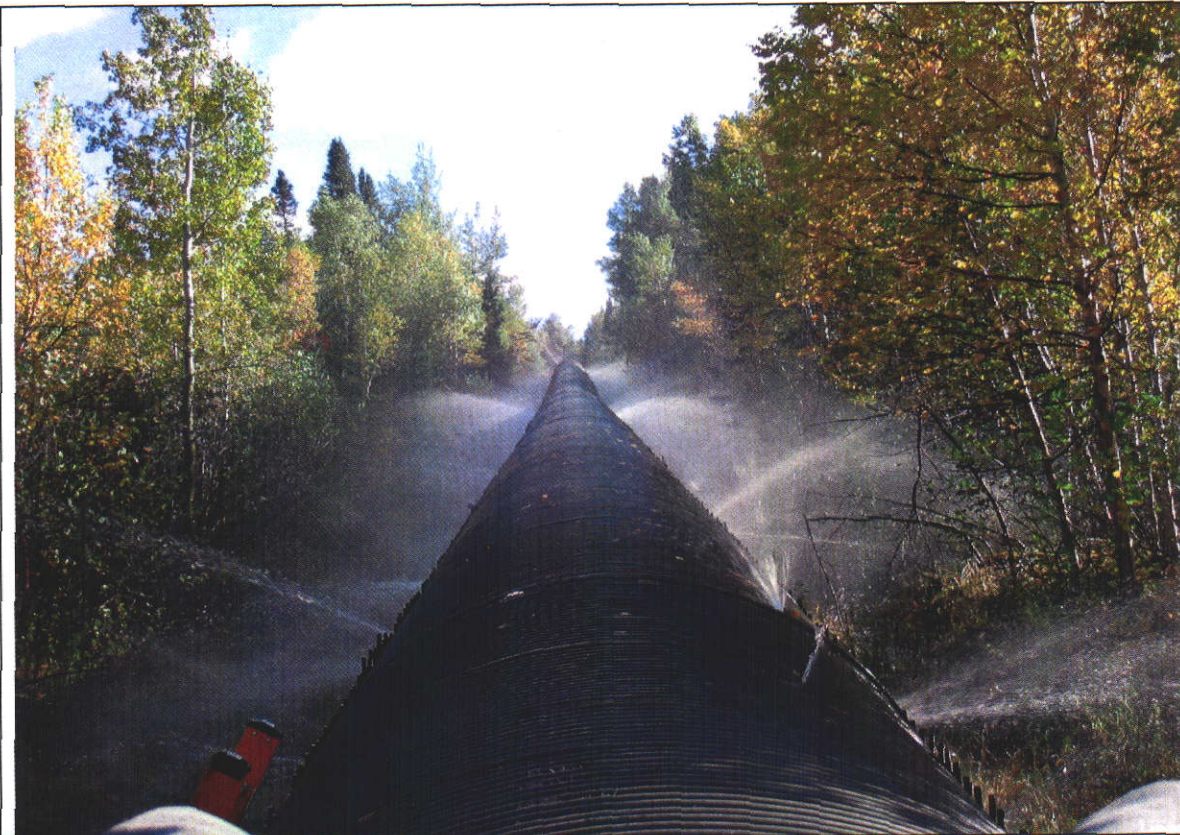
19. Wood stave penstock leakage.
