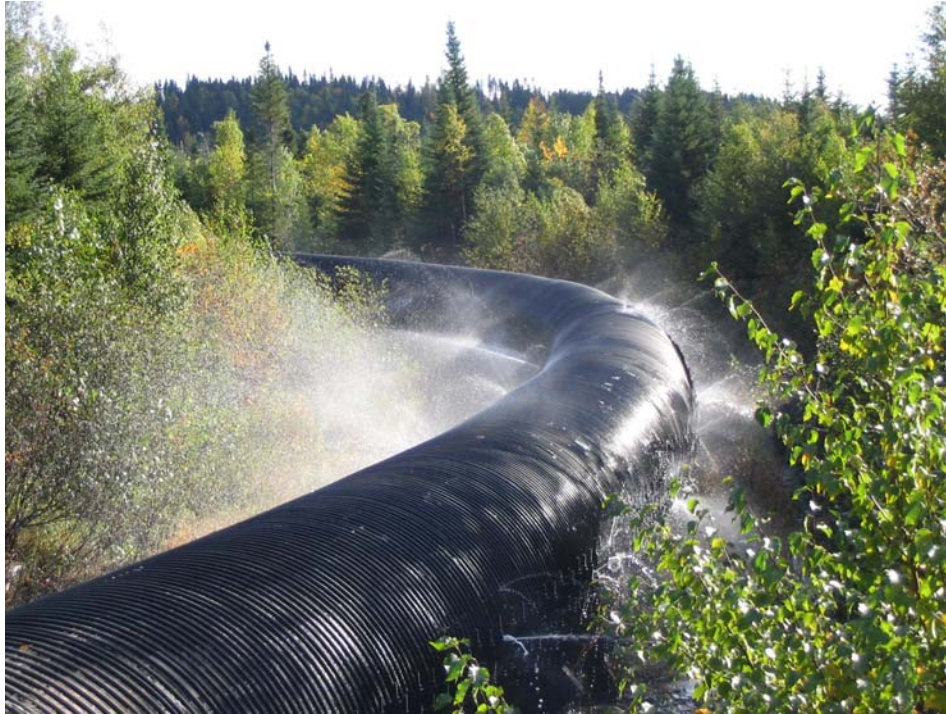
Figure 5: Water Leakage from Penstock
