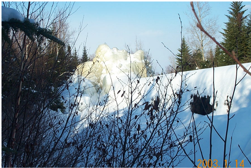
Figure 9: Ice Build-up on Penstock due to Water Leakage
