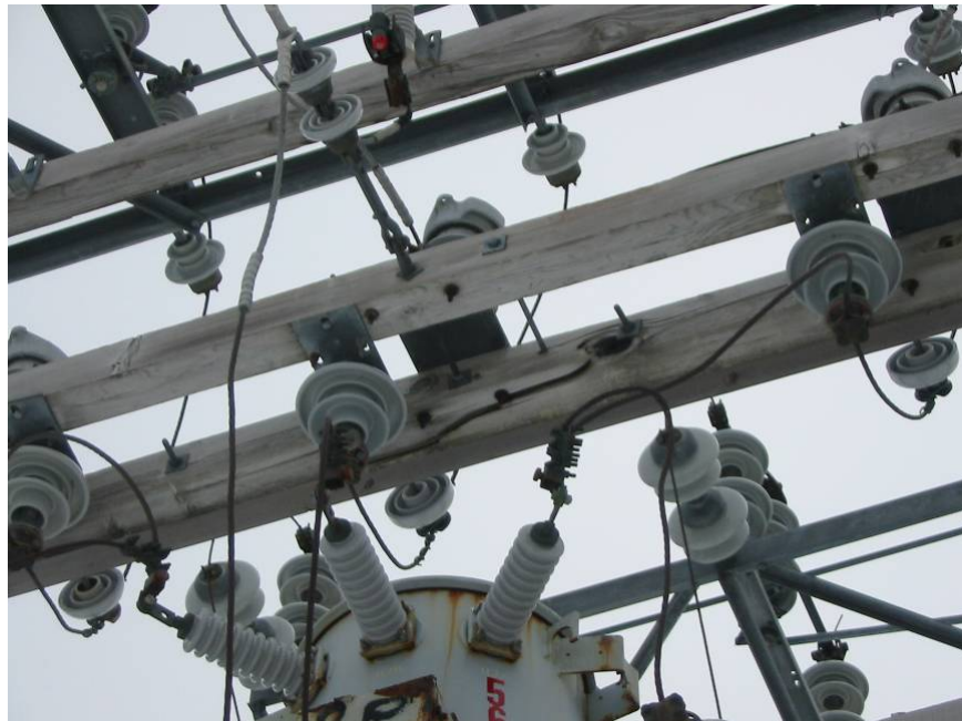
Cracked crossarm Garnish Substation
