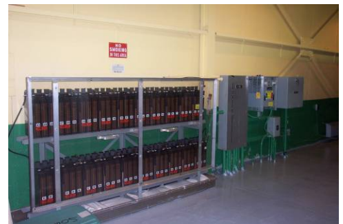
Figure 3 - Battery Bank
