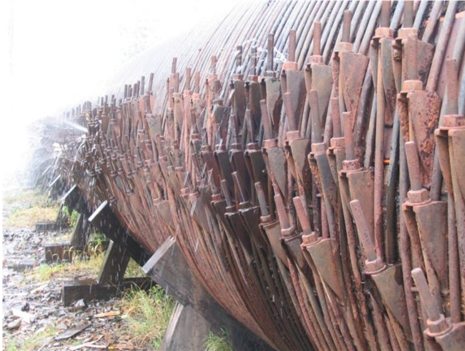
Figure 16: Leakage at Lower Section of Penstock
