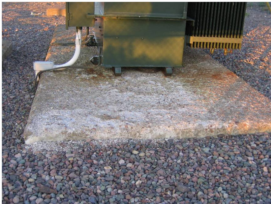
Foundation damage Garnish Substation
