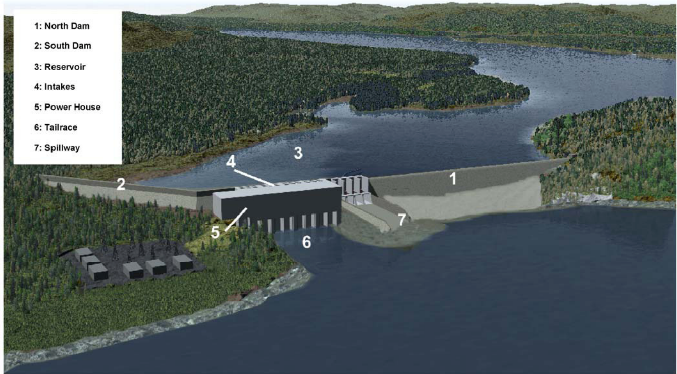
Figure 4-3 Conceptual Layout of Muskrat Falls Generation Facility
