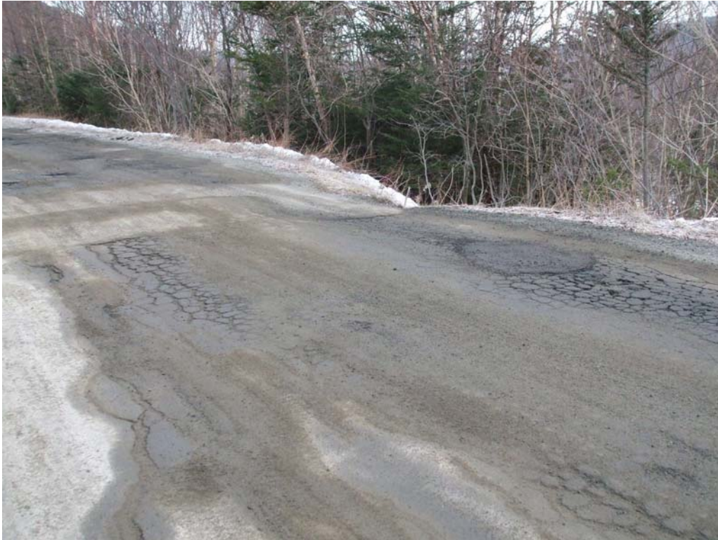
Figure 2: Road Damage Caused by a Collapsed Cross-Culvert
