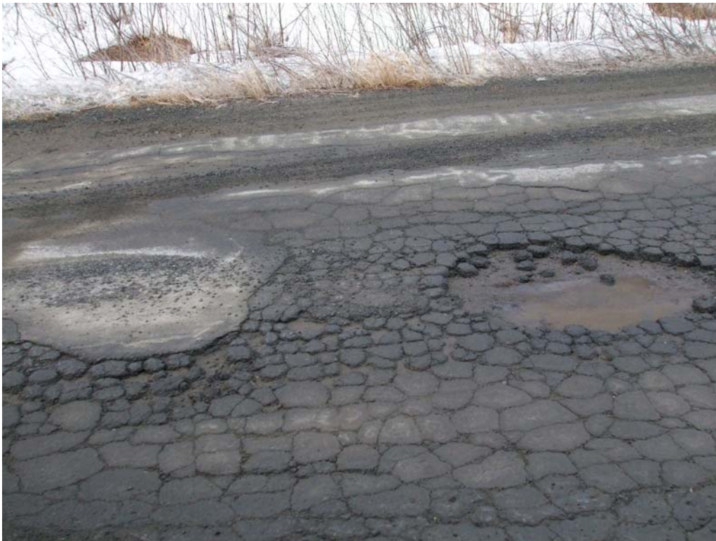
Figure 1: Road Structural Failure due to Trapped Water
