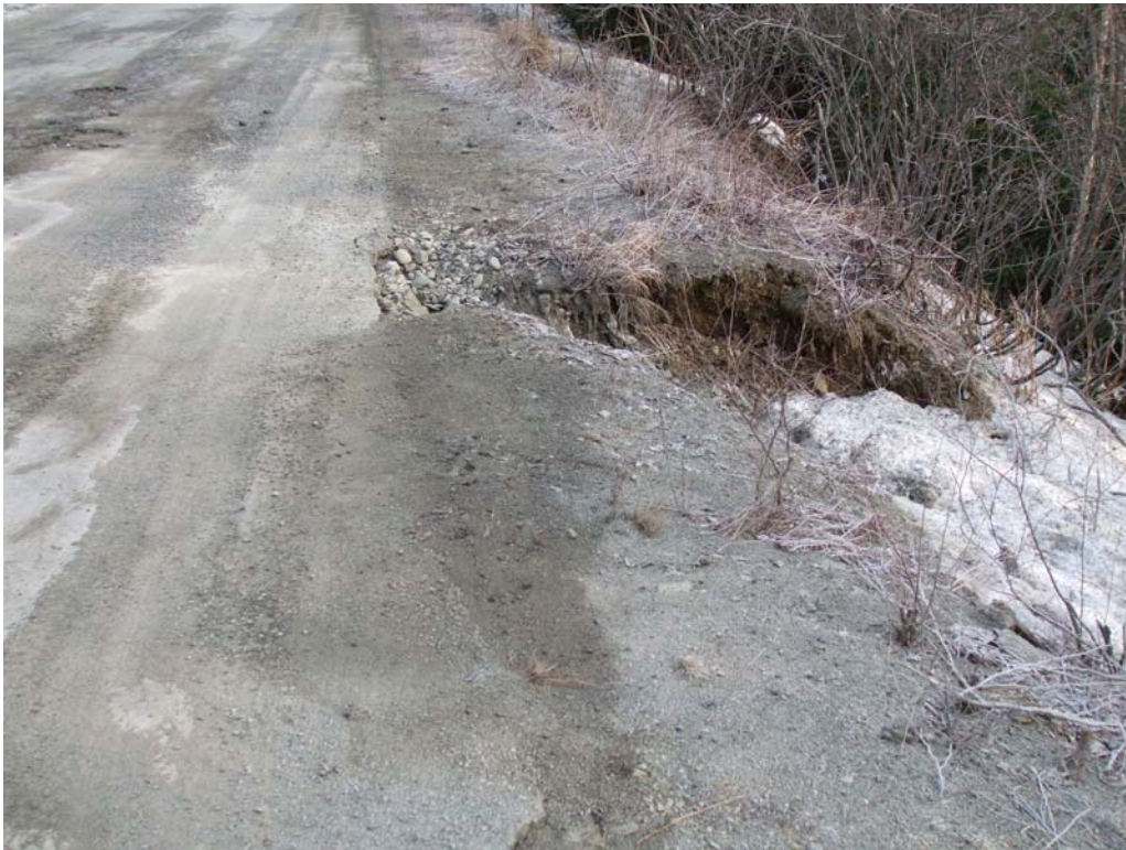
Figure 3: Erosion of the Shoulder of the Road
