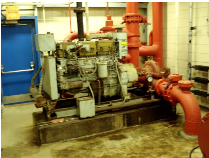
Figure 1: Diesel Fire Pump
