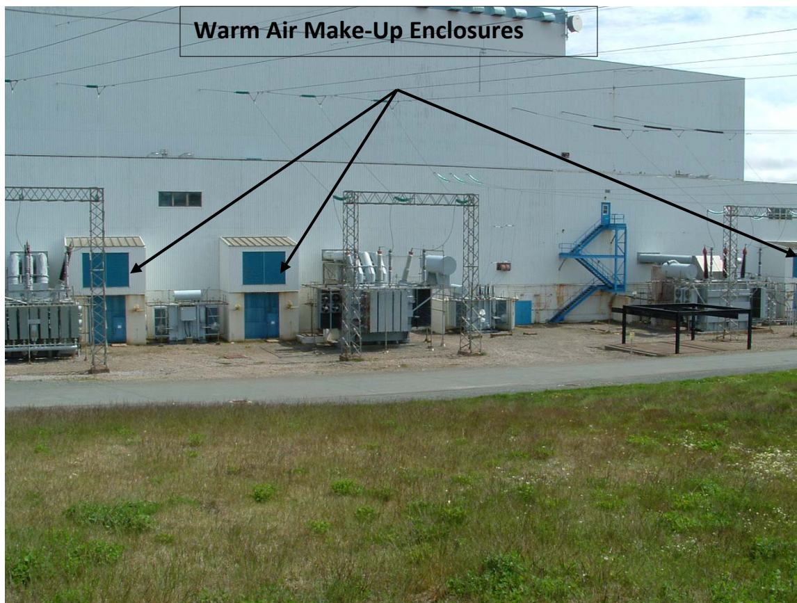
Figure 1 - Warm Air Make-Up Enclosures, South Side of Power House.
