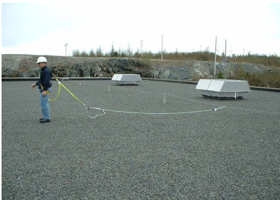
Figure 1: Roof Fall Protection System
