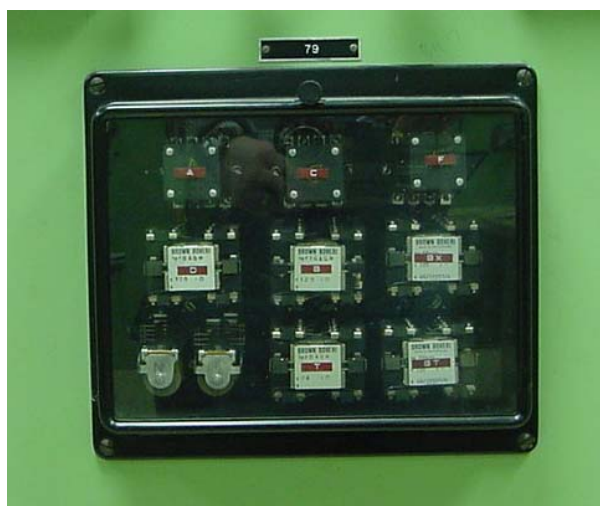
Figure 1: Discontinued Electromechanical Relay
