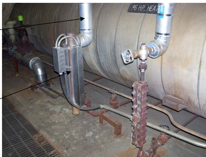
Figure 2 – HP Heater Level Probe
