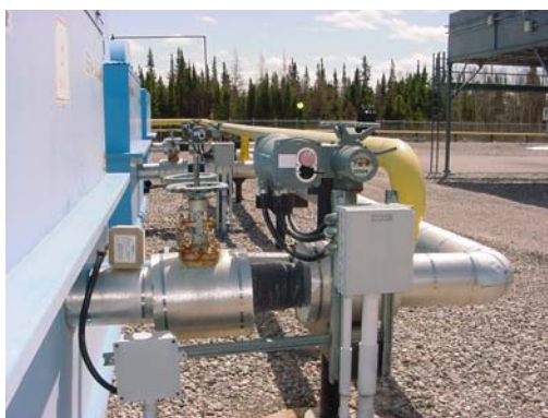
Figure 4: Fuel tank valve, actuation and associated junction box
