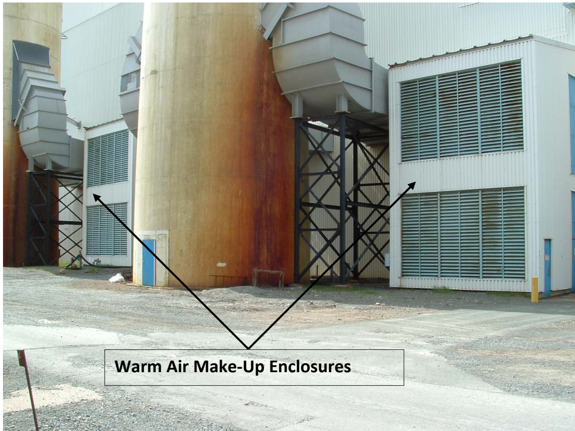
Figure 2 - Warm Air Make-Up Enclosures, North Side of Power House.
