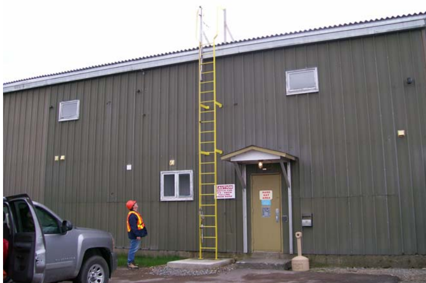
Figures 2 and 3: Ladder Fall Protection System
