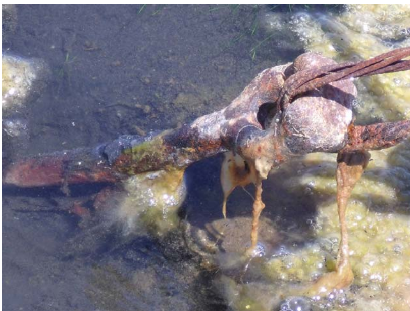
Figure 2: Corroded anchor rod (Typical)
