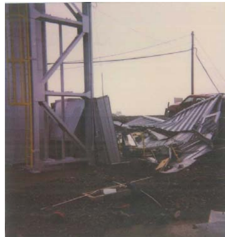
Figure 3. Intake Gate 2 Destroyed in July 2000
