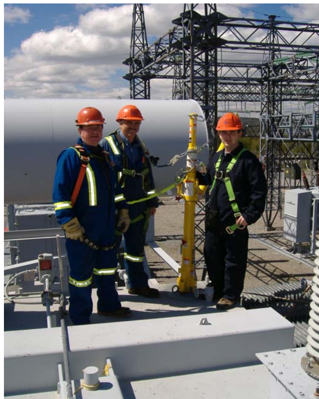
Figure 4: Transformer Fall Protection System
