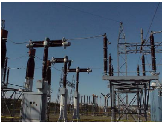
Figure 2: Breaker Failure Due to Moisture Ingress at the Hardwoods Terminal Station.
