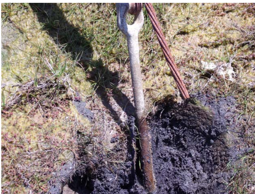
Figure 1: Corroded anchor rod (Typical)
