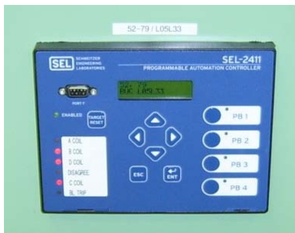
Figure 2: Microprocessor Based Relay
