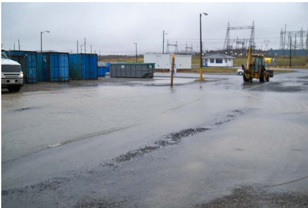
Figure 1: East Side of Powerhouse, December 2008. 250mm of Standing Water Covering Entire Road.
