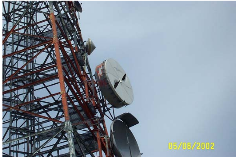
Figure 3: Heavily Damaged Radome
