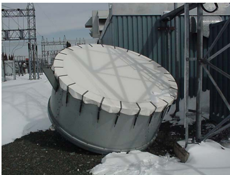
Figure 1: Microwave Antenna with Radome
