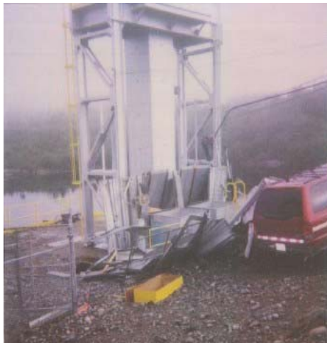
Figure 3. Intake Gate 2 Destroyed in July 2000
