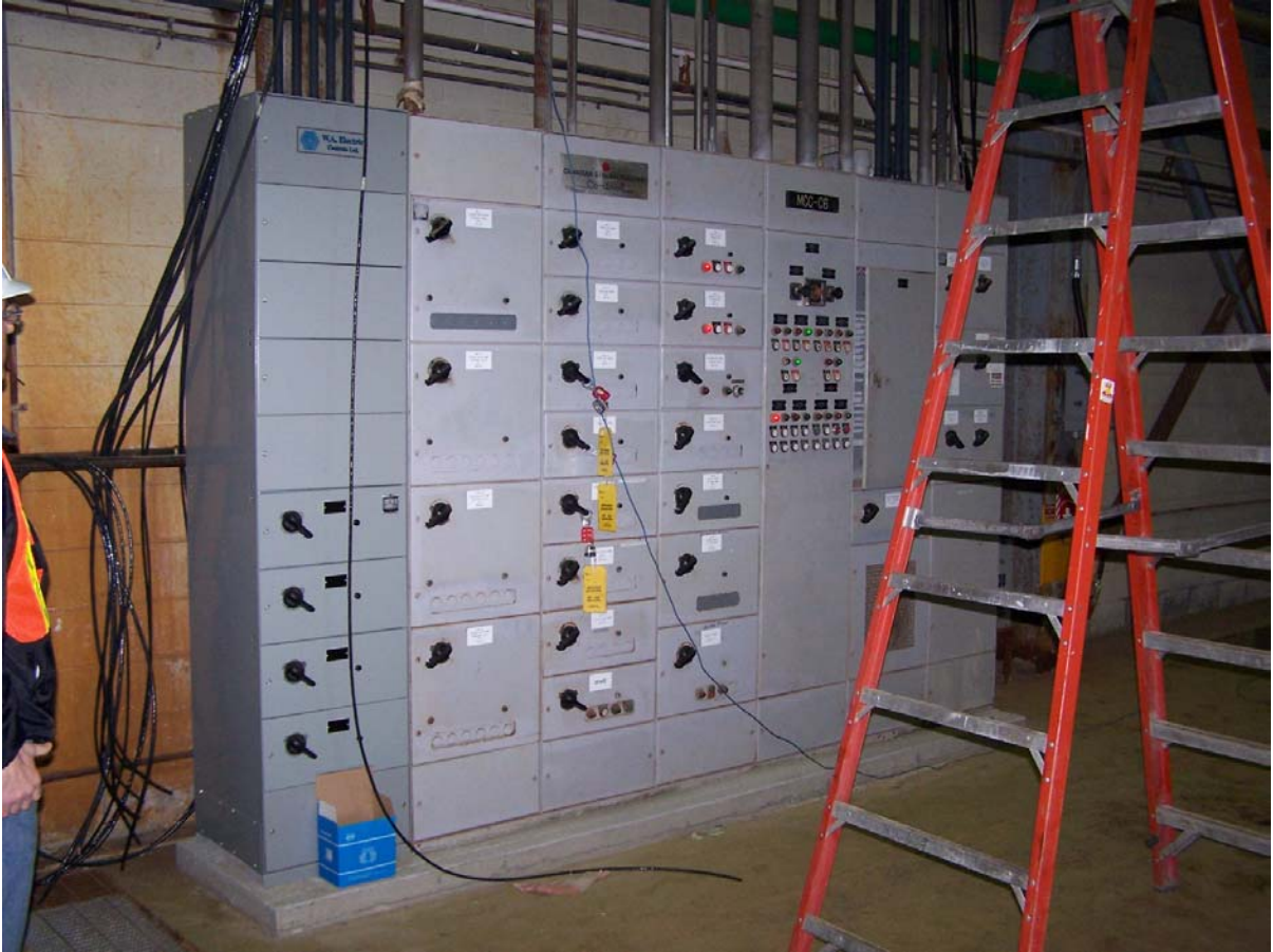
Figure 1: Motor Control Center in Pumphouse 1
