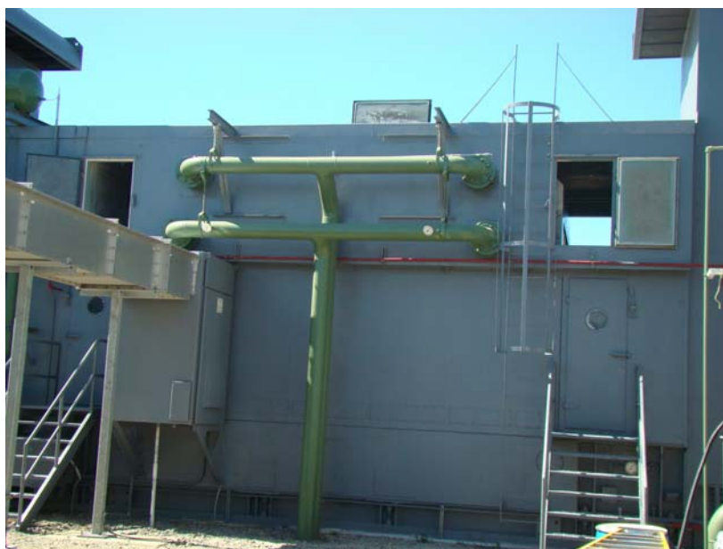
Figure 5: Alternator Enclosure – Emergency Doors Open
