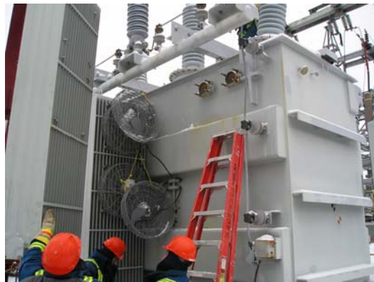
Figure 4: Radiators Being Replaced at Bottom Waters
