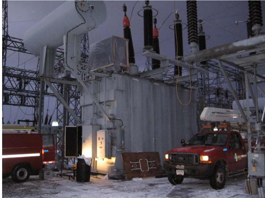
Figure 1: Power Transformer T3 at Massey Drive
