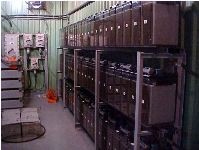
Figure 1 - Flooded-cell battery (Stephenville)
