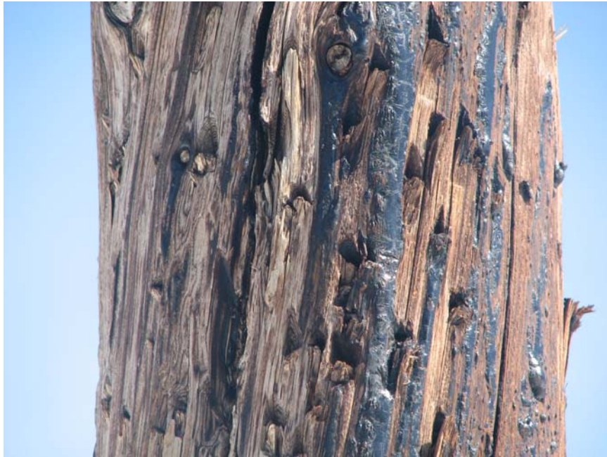
Figure 3: Typical deteriorated pole (Blackjack).
