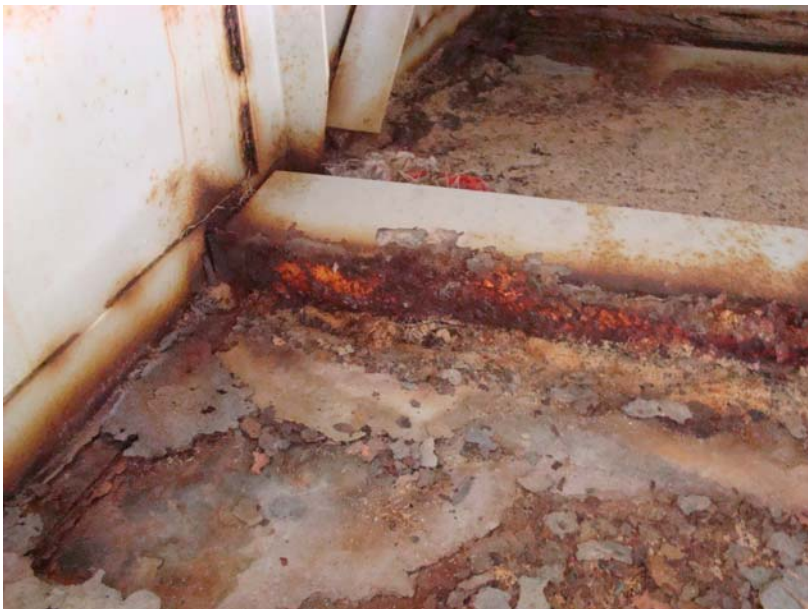
Figure 4: Inside View of Wind Box - Alternator Glycol Cooler
