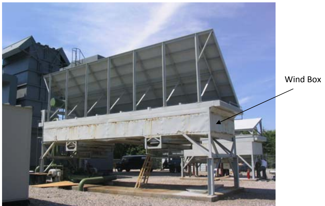
Figure 2: Alternator Glycol Cooler
