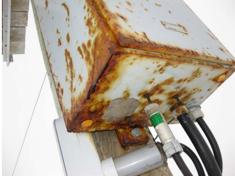
Figure 2: Shoal Cove N Recloser Control Cabinet
