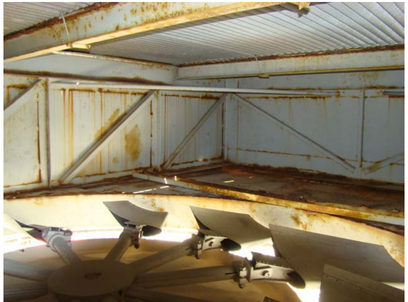
Figure 3: Inside View of Wind Box – Alternator Glycol Cooler
