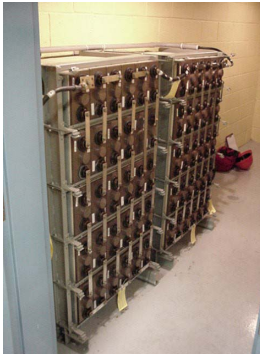
Figure 2 - VRLA battery (Hinds Lake)
