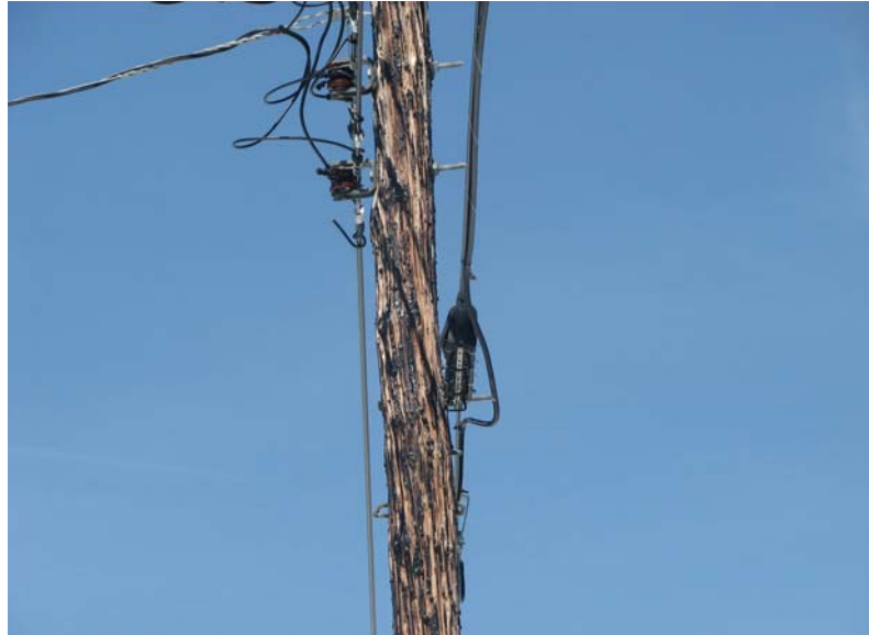
Figure 1: Typical Blackjack Wood Pole Structure
