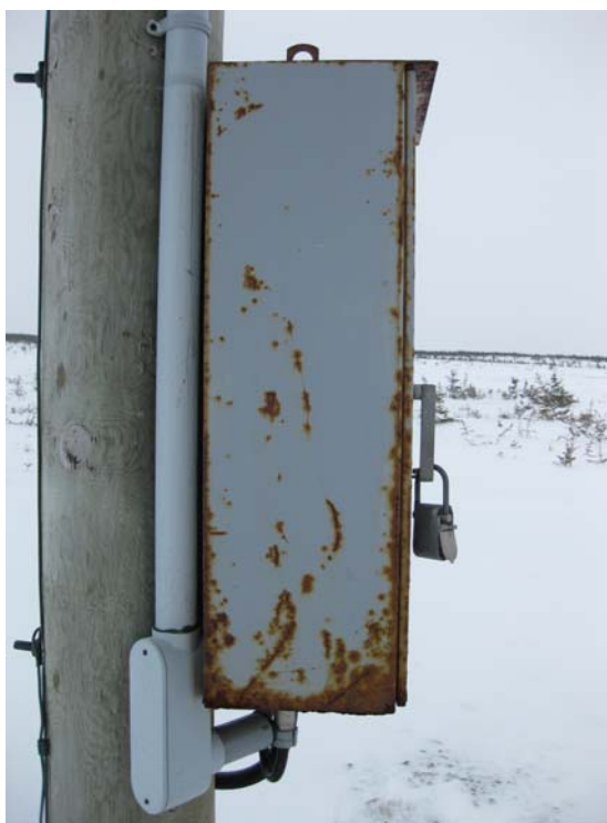
Figure 1: Shoal Cove N Recloser Control Cabinet
