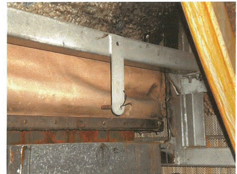
Figure 5 Expansion joint belt in good condition.
