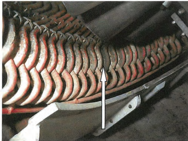
Discoloration heating pattern on some coils.
