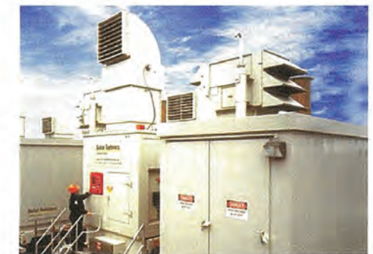
Sited Configuration of Mobile Power Unit
