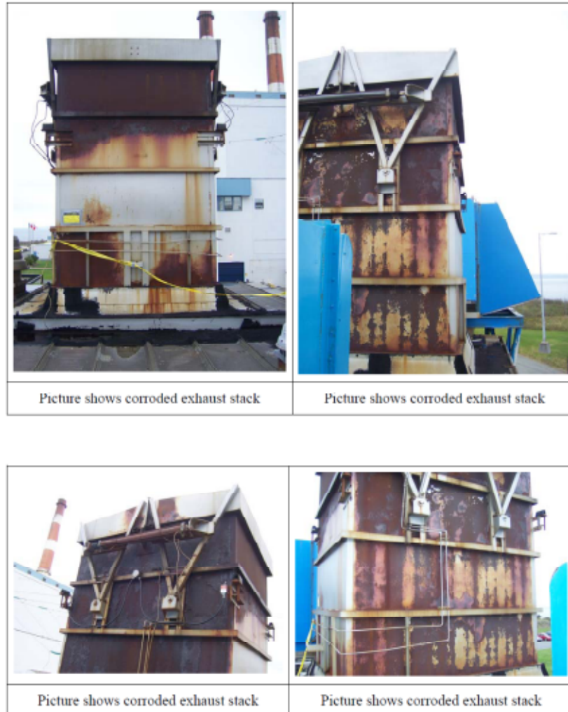
FIGURE 2-7 CORRODED EXHAUST STACK (GAS TURBINE PLANT)
