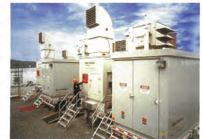
Sited Configuration of Taurus 60 Mobile Power Unit
