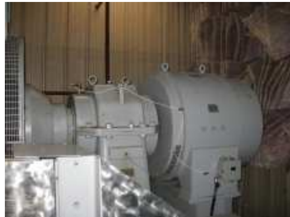
FIGURE 2-1 GTG GAS ENGINE & GENERATOR
