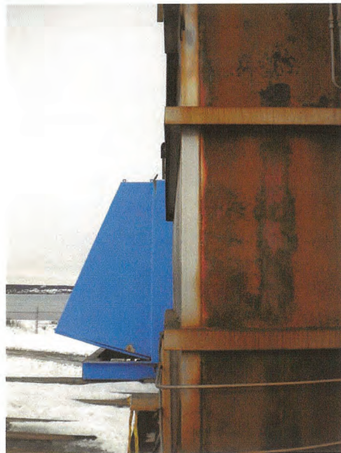
Figure 3 – Slight bulge in sidewall.
