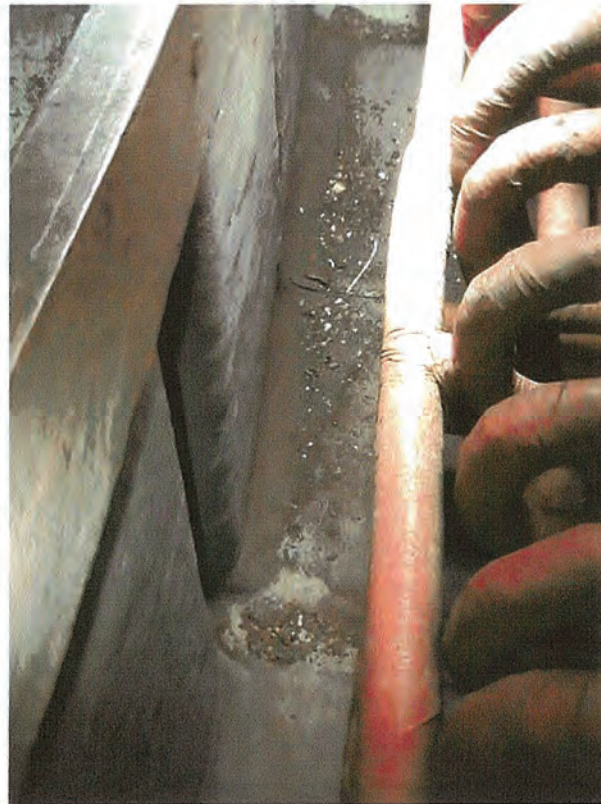
Rust flakes present in bottom of stator enclosure.
