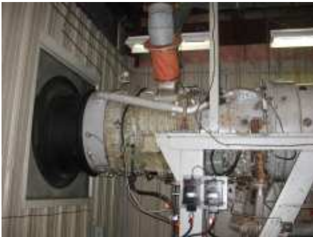
FIGURE 2-1 GTG GAS ENGINE & GENERATOR
