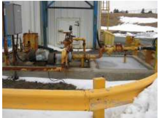
FIGURE 2-6 LIGHT OIL RECEIVING SYSTEM AND STORAGE TANKS
