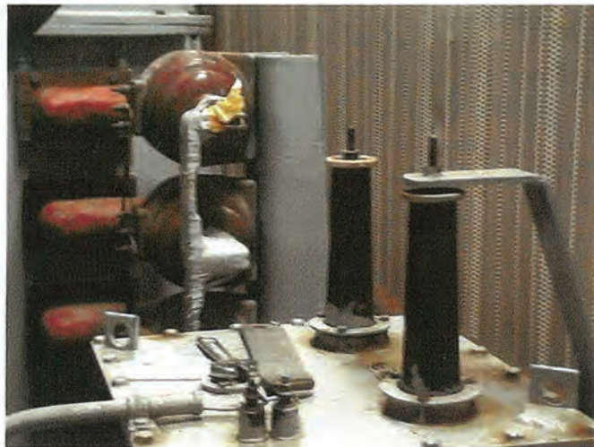
Star Point had to be disconnected from transformer for true reading. With this point connected insulation resistance to ground reading is 2000 \Omega .
