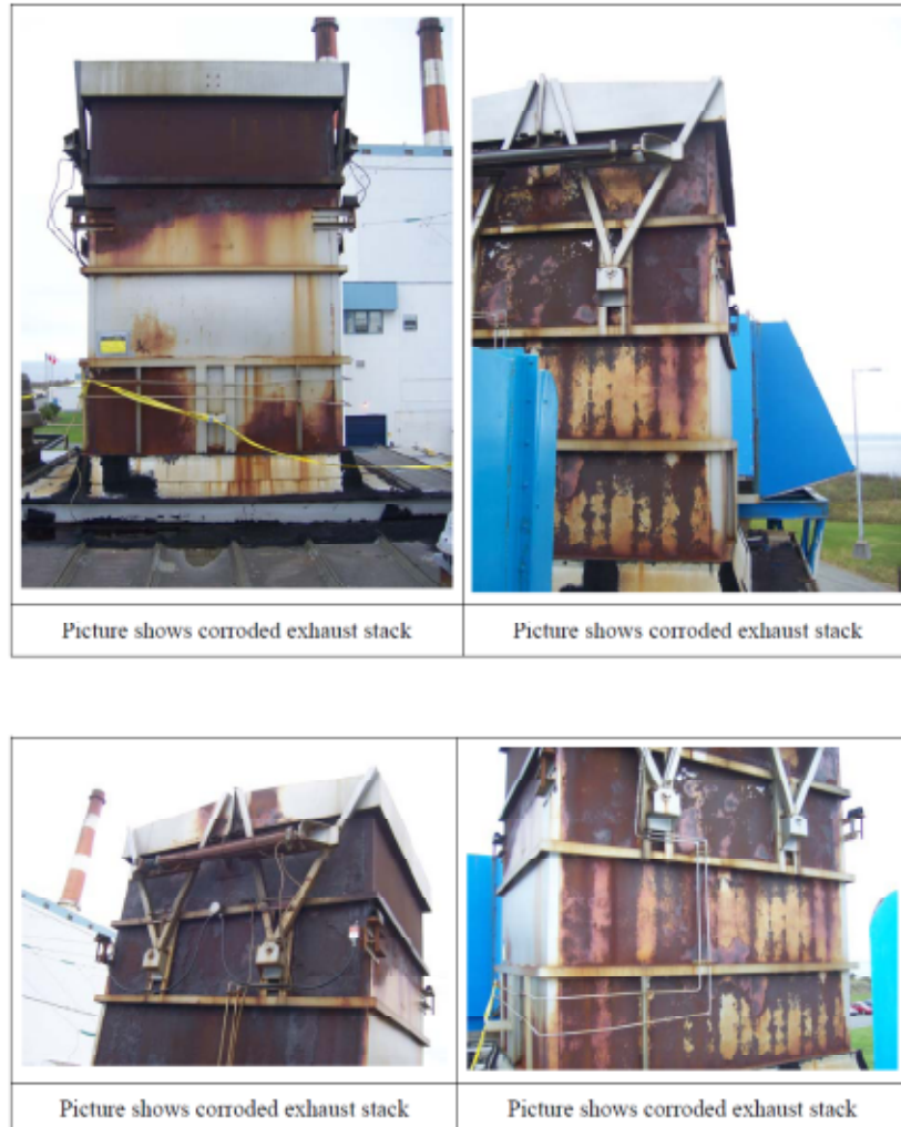
FIGURE 2-7 CORRODED EXHAUST STACK (GAS TURBINE PLANT)
