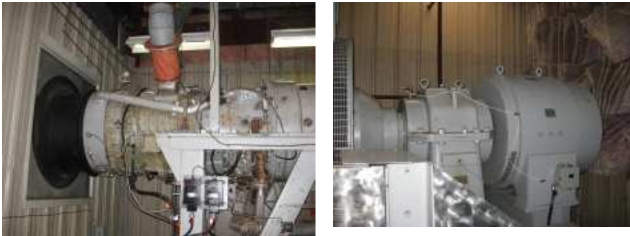
FIGURE 2-1 GTG GAS ENGINE & GENERATOR
