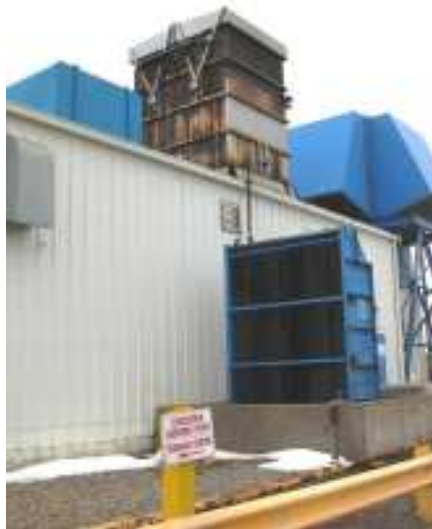
FIGURE 2-4 LIGHT OIL RECEIVING & LUBE OIL RADIATOR
