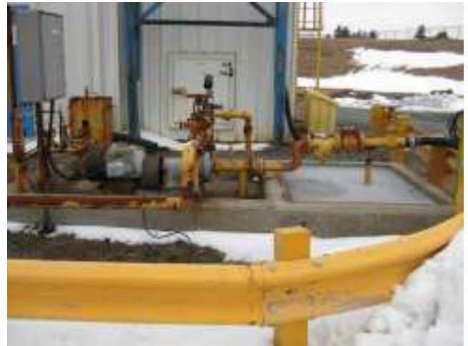
FIGURE 2-6 LIGHT OIL RECEIVING SYSTEM AND STORAGE TANKS
