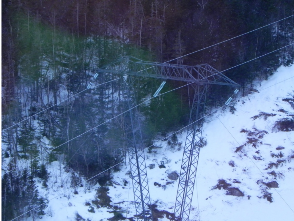
Figure 2-9a: Picture of TL217 Structure 282 with Damaged Insulators
