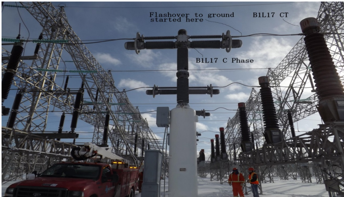
Figure 2-5a: Holyrood Breaker - B1L17 C Phase
