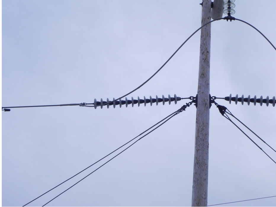
Figure 2-13b: TL201 Structure 210 Right Phase Jumper
