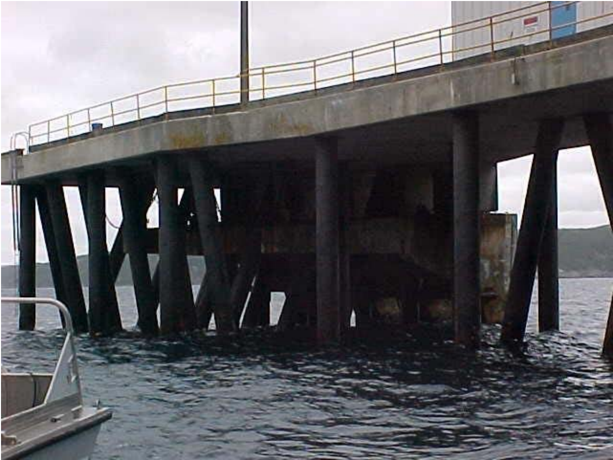
Figure 6: Jetty Pile System
