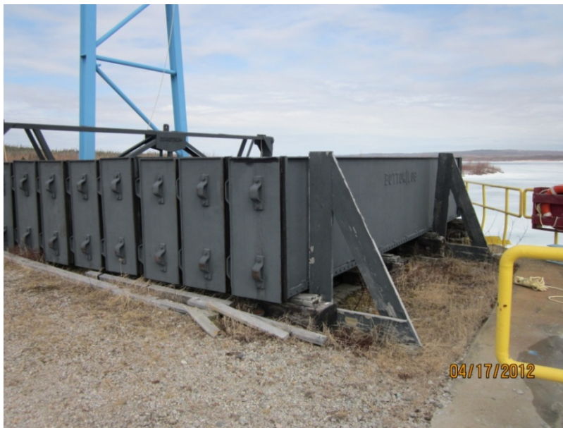
Figure 2: Burnt Dam Stop Logs – Current Storage Arrangement
