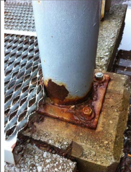
Photo #15: Ground Connection on Stair
