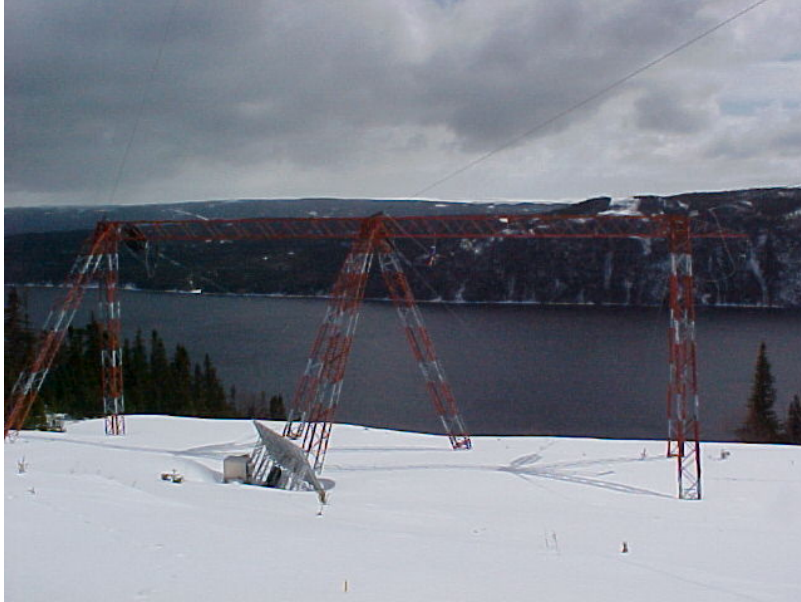
Figure 2: Site #1 crossing structure
