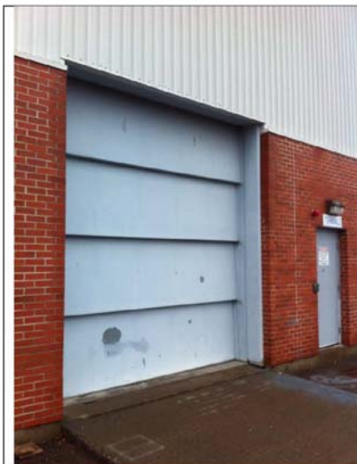
Photo #11: Overhead Accordion Door
