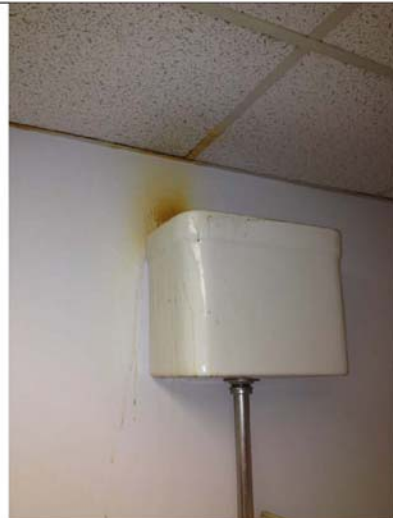
Photo #20: Urinal tank
