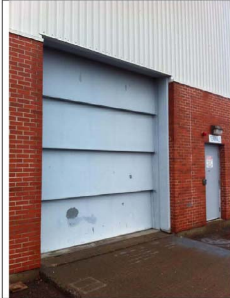
Photo #11: Overhead Accordion Door
