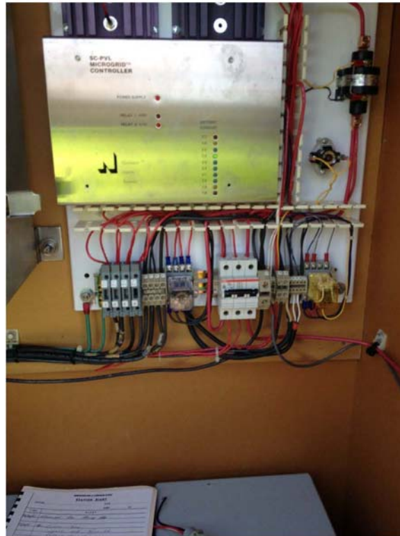
Figure 5 - System Controller
