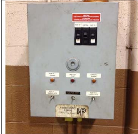
Photo #23: Duplex Oily Water system
