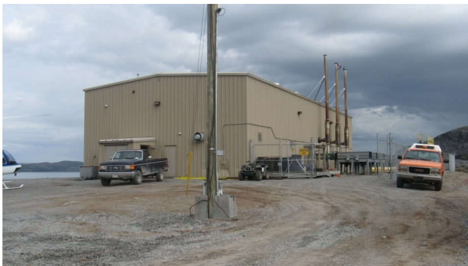
Figure 1: Nain – Diesel Generating Plant.
