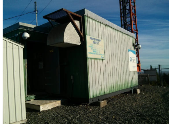
Figure 3: Weathered Siding
