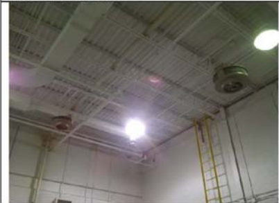
Photo #29: Metal Halide High Bays
