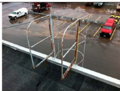
Photo #14: Roof Access
