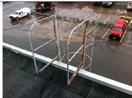
Photo #14: Roof Access
