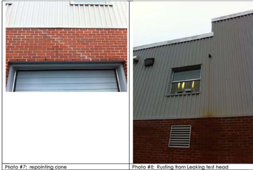
Photo #7: repointing cone
