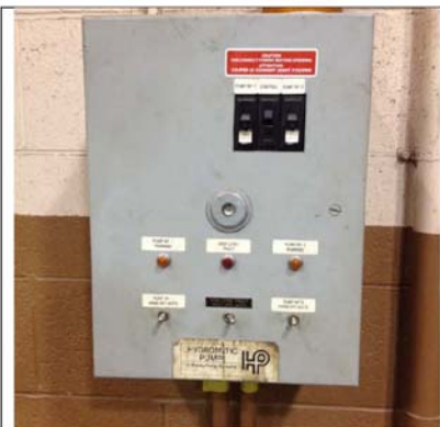
Photo #23: Duplex Oil Water system
