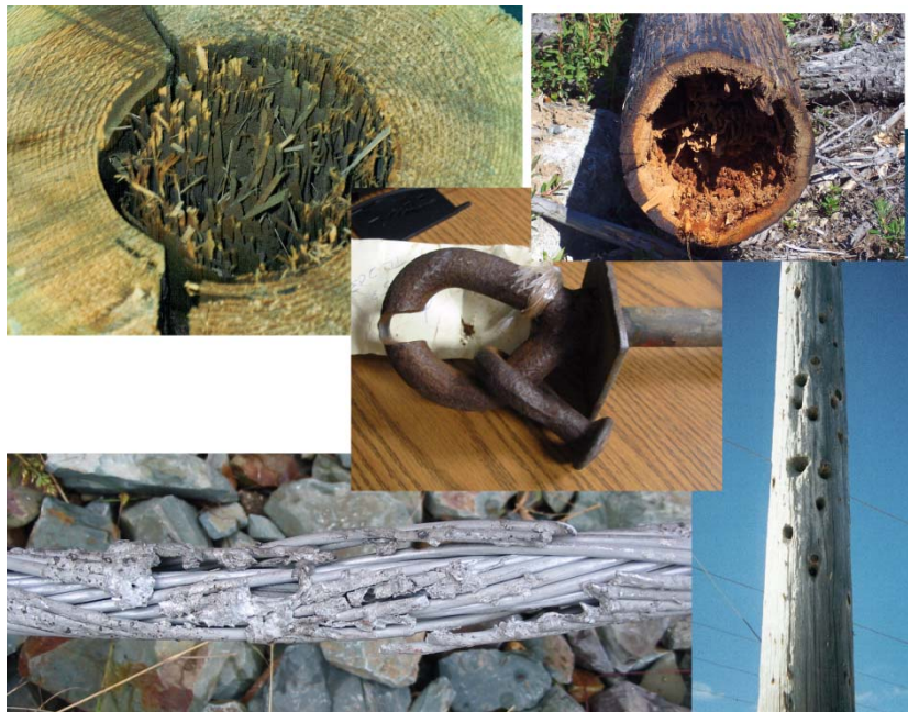
Figure 2: Typical Wood Pole Inspection Results
