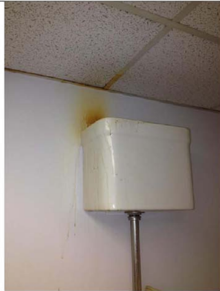
Photo #20: Urinal tank
