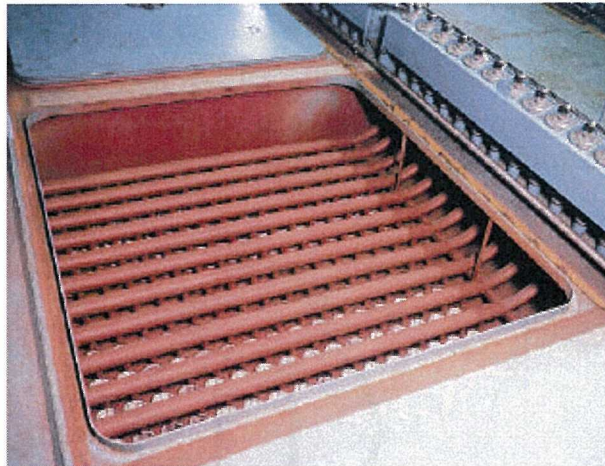
Typical LKP Nozzle Pipe Assembly
