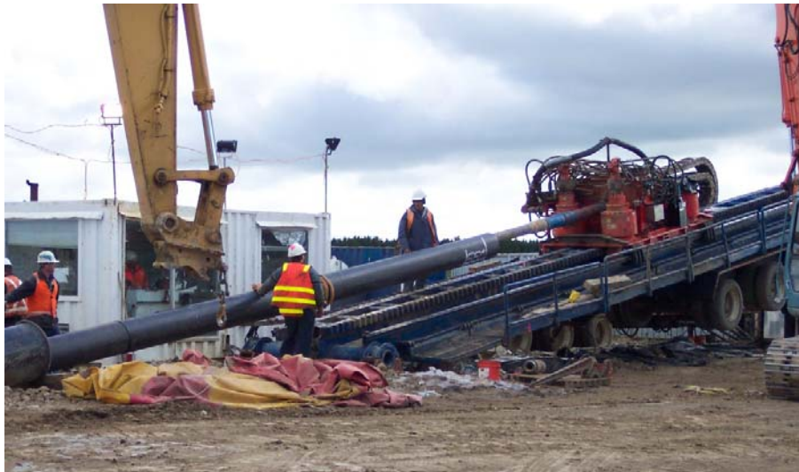
Figure 2-12: Photograph of Drilling Rig Pushing in HDPE Casing Pipe
