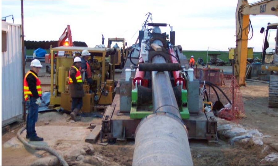
Figure 2-14: Photograph of Thruster Installing Casing Pipe
