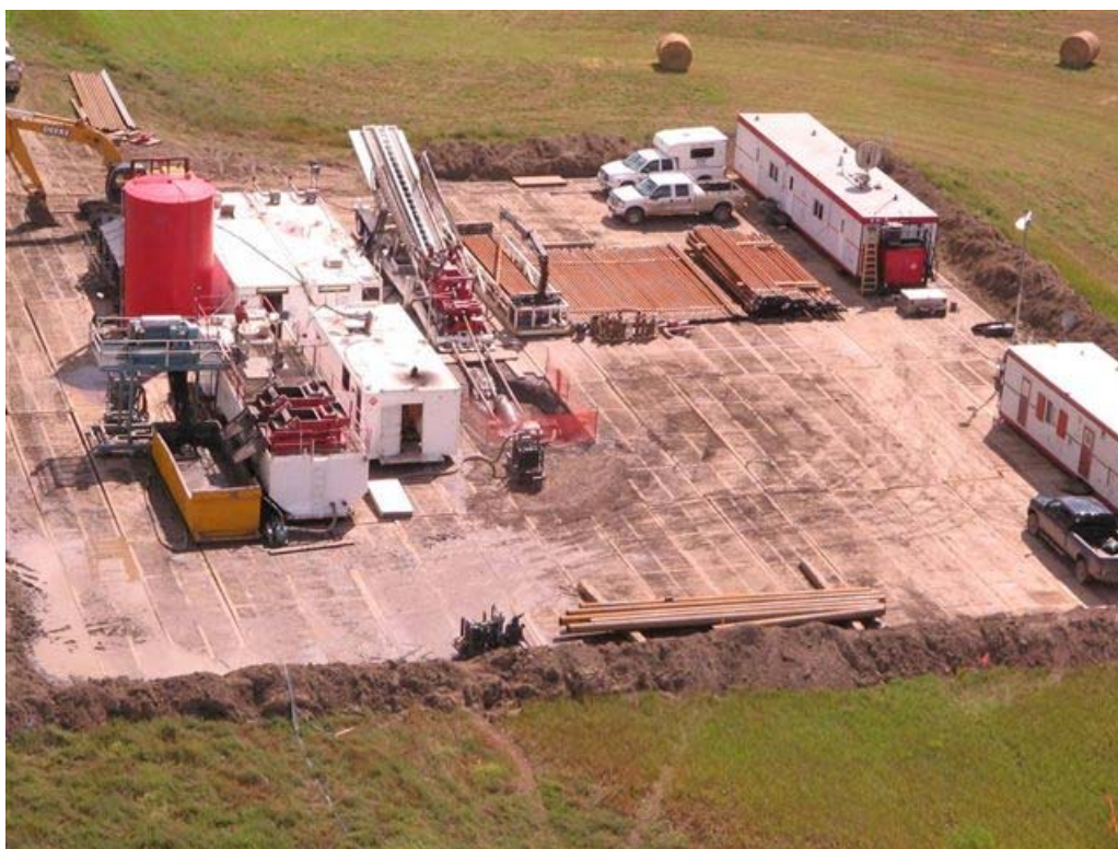
Figure 3-1: Typical Large Diameter HDD Entry Location Setup
