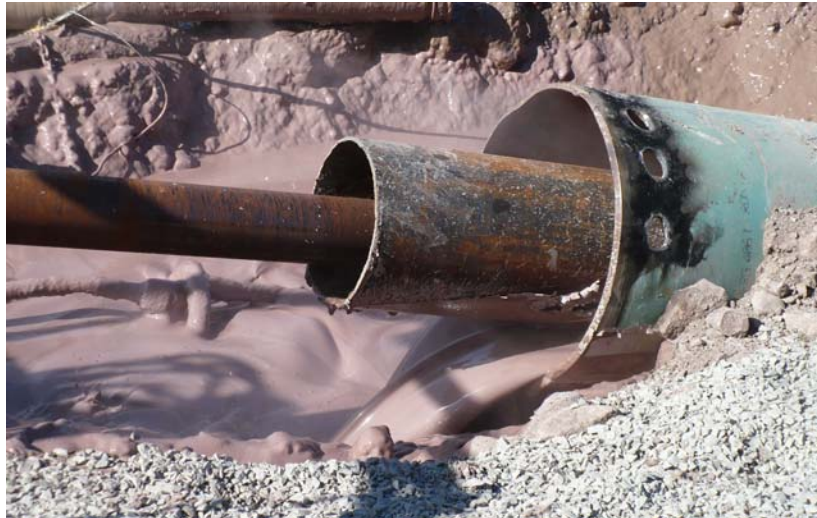
Figure 2-3: Photograph of Typical Drilling Fluid Returns at Drill Rig Location
