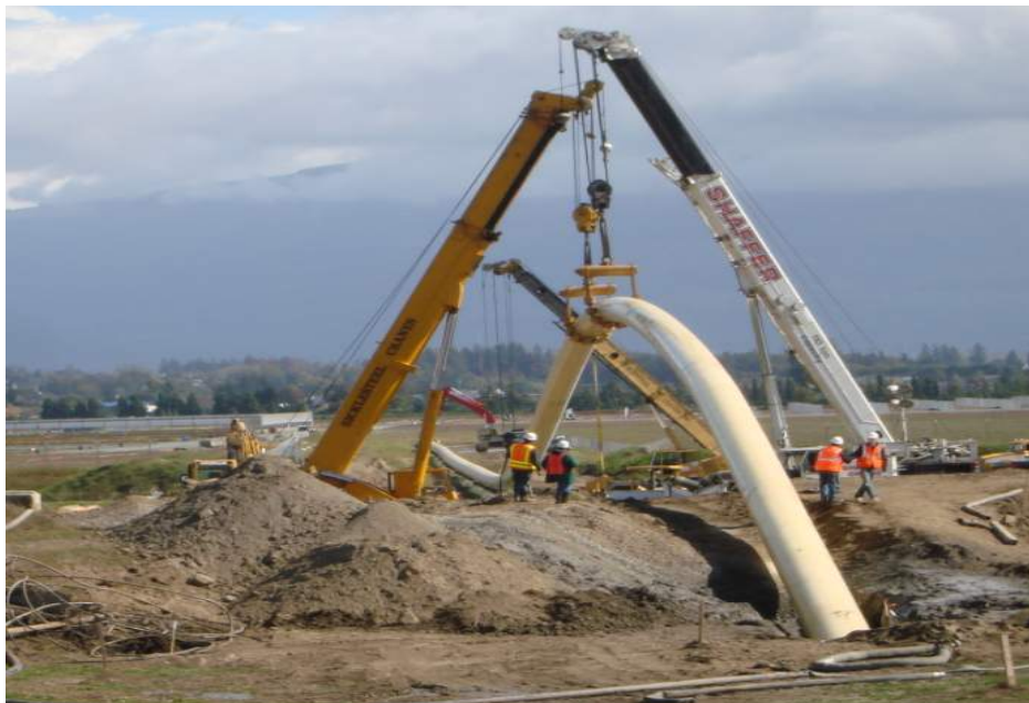
Figure 2-11: Photograph of Steel Pipeline Insertion with Pullback Towards Drill Rig
