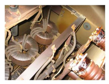
In order to access any further test points the core would have to be removed. To accomplish this we would have to remove the top cover, let go the secondary & tertiary
