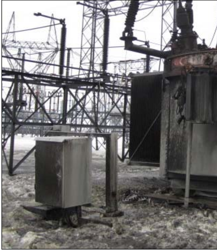
Figure 7: Sunnyside Station Service Transfer Switch
