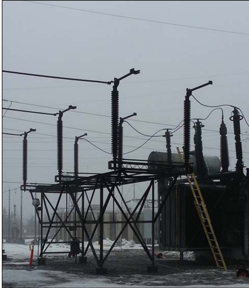
Figure 6: Sunnyside 230 kV B1T1 Disconnect Switch
