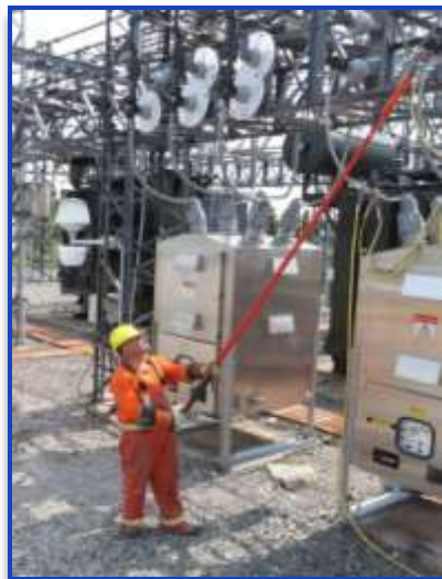
Newfoundland Power employee completing substation switching
