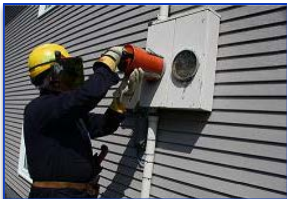
Installation of a replacement AMR meter
