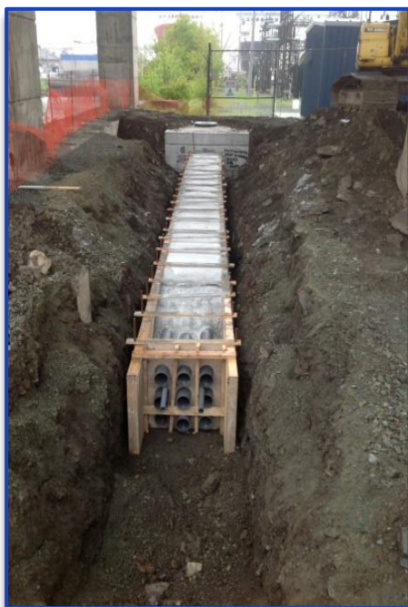
New duct bank near the St. John's Main Substation along the banks of the Waterford River.
