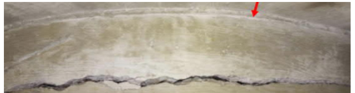
Figure 5-17: Unit 3 South Sump Crack in East Beam
