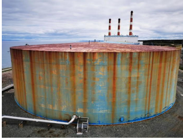
Figure 5-61: HFO Tank 2 with Deteriorating Coating
