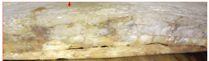
Figure 5-13: Unit 2 South Sump Crack in West Beam
