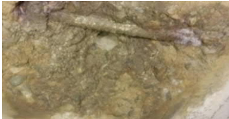
Figure 5-27: Unit 1 North East Sump - Exposed Rebar North End of Sump
