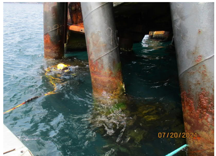
Figure 5-53: Typical Corrosion Present at Water Line on Jetty Piles (Piles 29B, 29C, 29D Jetty South End)
