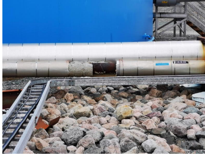
Figure 5-6: Auxiliary Steam Line in Tank Farm Facility Observed with Insulation Removed
