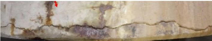
Figure 5-30: Unit 1 South Sump - Crack in Ceiling Near Southwest Access Point
