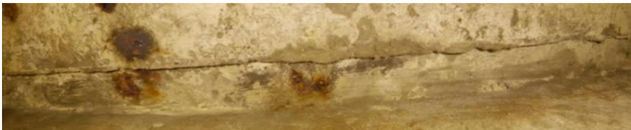
Figure 5-28: Unit 1 North East Sump - Crack in Ceiling Along West Wall
