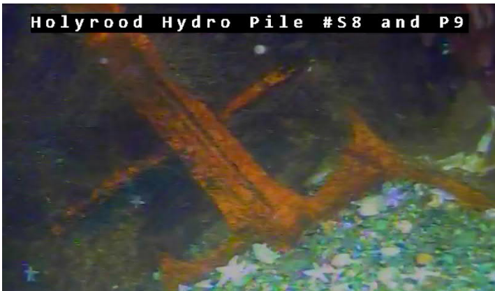
Figure 5-58: Pile P9 Concrete Jacket completely Deteriorated beneath the Water Line. Typical for Pile S8 and P9
