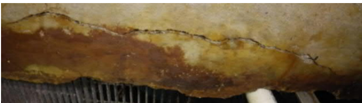
Figure 5-44: Unit 3 South Sump - Crack in Ceiling Near North Access Grating
