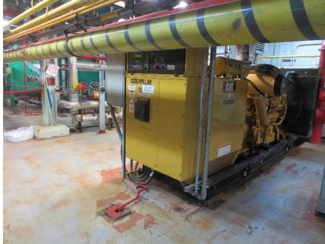
Figure 5-3: Emergency Genset in Powerhouse
