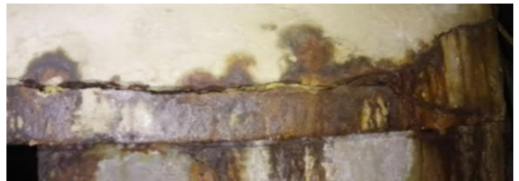
Figure 5-20: Unit 4 South Sump Crack in West Beam
