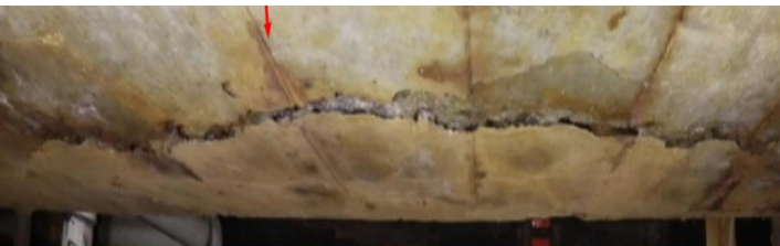
Figure 5-32: Unit 1 South Sump - Crack in North End Beam
