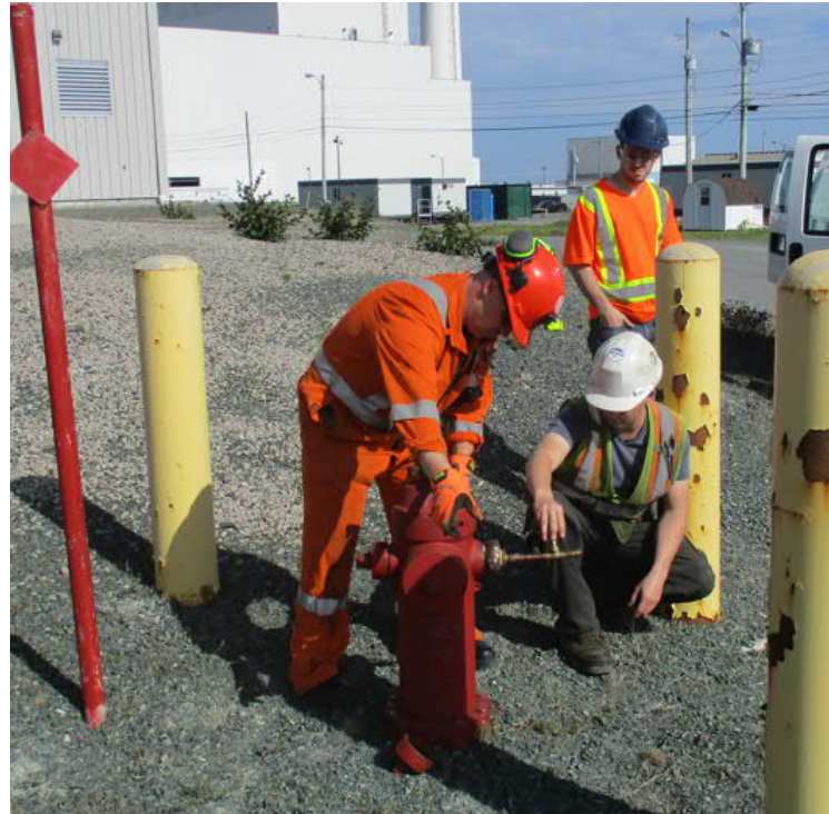
Figure 7-1: Static Testing on Firewater Hydrant Northeast of CT Building
