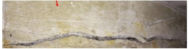
Figure 5-15: Unit 3 South Sump Crack in East Beam
