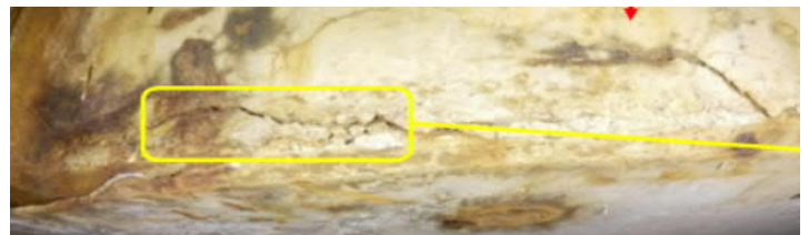
Figure 5-47: Unit 4 North West Sump - Crack Near South Access Grating
