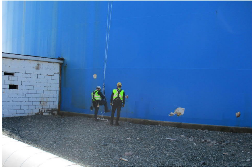
Figure 5-62: Fuel Tank #3 North Quadrant Localized Paint Deterioration
