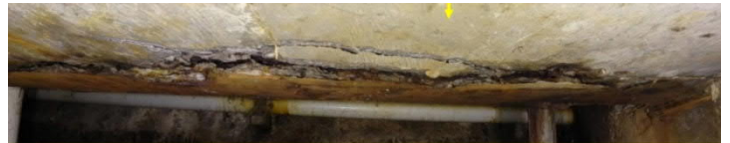
Figure 5-31: Unit 1 South Sump - Crack in Ceiling in Center of Sump
