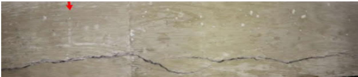
Figure 5-18: Unit 3 South Sump Crack in East Beam
