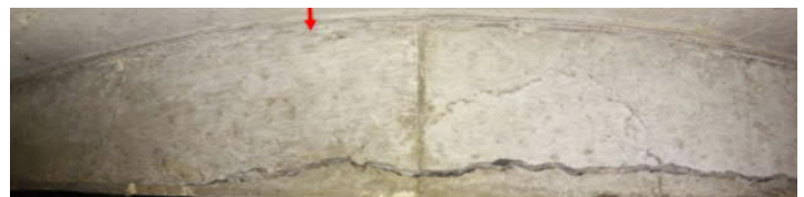
Figure 5-11: Unit 1 South Sump Crack in East Beam
