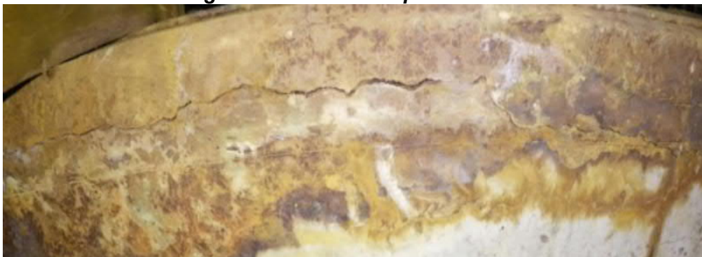
Figure 5-24: Unit 1 North West Sump – Crack on East Side
