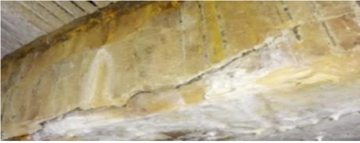
Figure 5-34: Unit 2 North West Sump - Crack Near South Stop Log Guides
