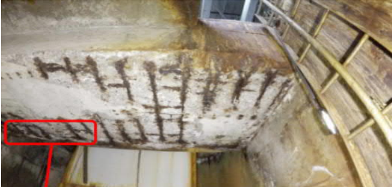
Figure 5-23: Unit 1 North East Sump: Exposed Rebar Near Access Point
