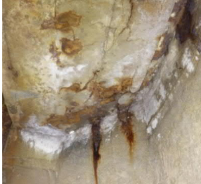
Figure 5-29: Unit 1 North East Sump: Deterioration of Concrete in Ceiling Near Traveling Screens
