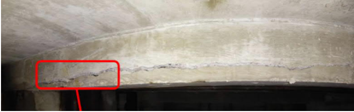
Figure 5-14: Unit 3 South Sump Crack in East Beam
