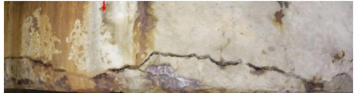
Figure 5-39: Unit 2 South Sump - Crack in Beam Near Southwest Access Point
