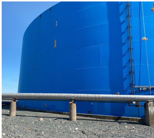
Figure 5-65: No. 3 Fuel Tank Southwest Quadrant Localized Paint Deterioration
