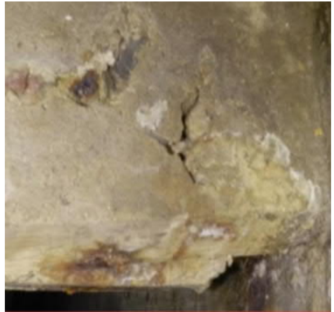
Figure 5-26: Unit 1 North West Sump - Crack in Southwest Corner
