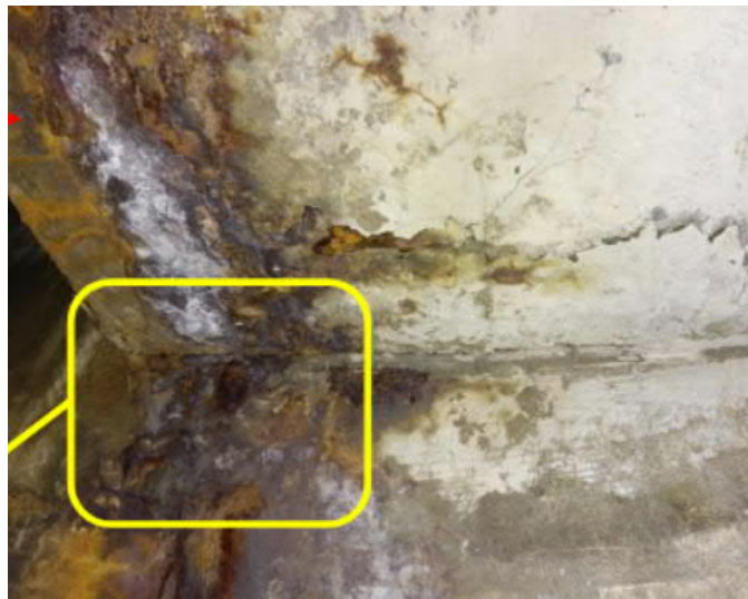
Figure 5-37: Unit 2 North East Sump - Deterioration in Southwest Corner
