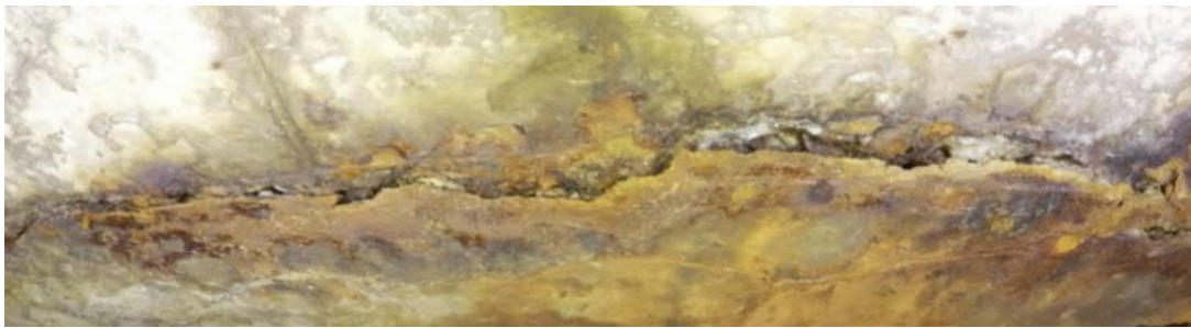
Figure 5-36: Unit 2 North East Sump - Crack in Ceiling Near Travelling Screen
