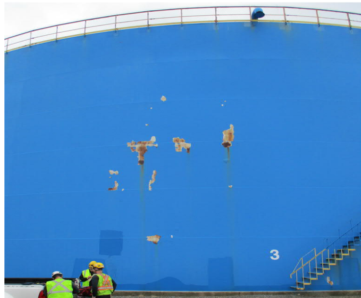
Figure 5-63: Fuel Tank #3 East Quadrant – Localized Paint Deterioration
