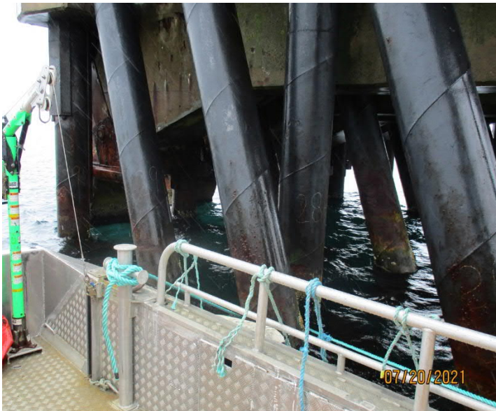
Figure 5-52: Typical Pile Condition Above Water Line (Jetty South End)
