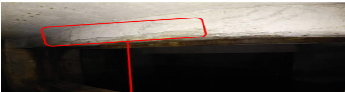
Figure 5-10: Unit 1 South Sump East Crack Location
