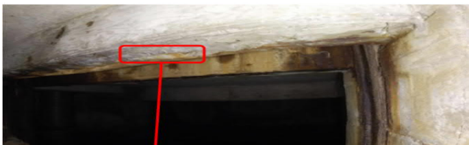
Figure 5-12: Unit 2 South Sump in West Beam Crack Location
