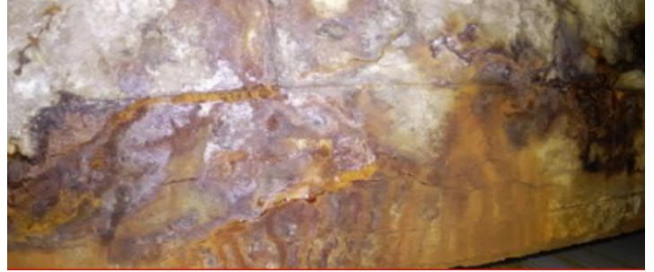
Figure 5-35: Unit 2 North West Sump: Deterioration of Concrete on Ceiling Near Travelling Screens
