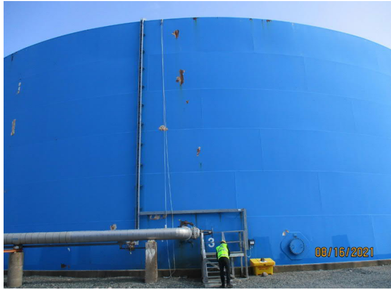
Figure 5-64: Fuel Tank #3 South Quadrant Localized Paint Deterioration
