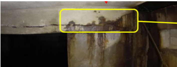
Figure 5-19: Unit 4 South Sump Crack in West Beam
