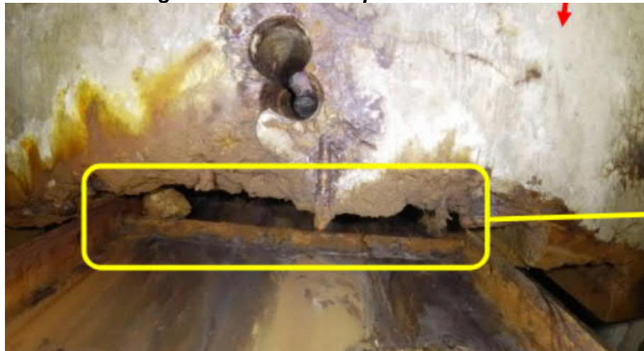
Figure 5-40: Unit 3 North West Sump - Deterioration in Ceiling Near Travelling Screen
