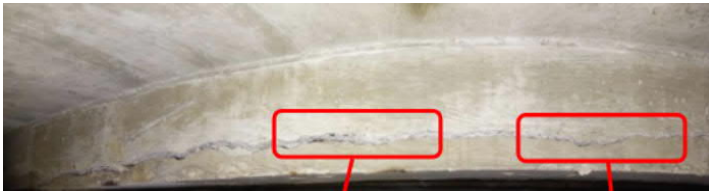
Figure 5-16: Unit 3 South Sump Crack in East Beam
