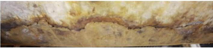
Figure 5-38: Unit 2 South Sump Crack in North End
