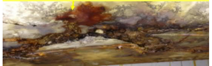
Figure 5-33: Unit 2 North West Sump - Deterioration of Ceiling Near South End
