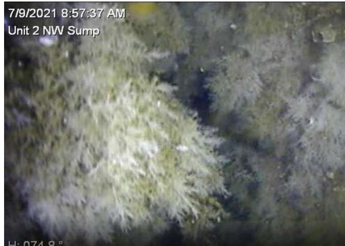
Figure 5-7: Marine Growth Found in Cooling Water Sumps (typical to All 4 Units)
