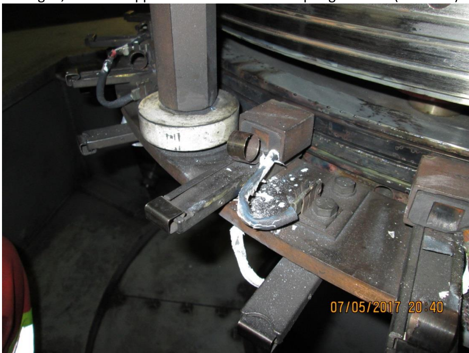
T7: The brush holder sides have holes melted in them, and some metal loss on the surface adjacent to the ring. The brush wear is at the threshold for replacement. The pigtail is melted off. (Pictures 8, 9 & 10)
