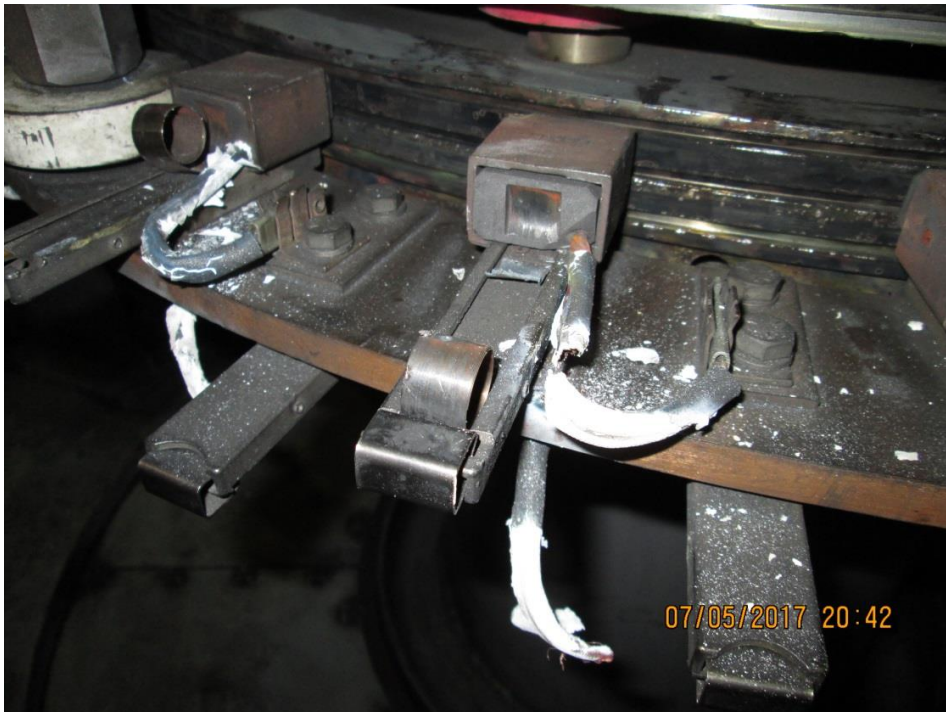
T6: The brush wear is at the threshold for replacement. The pigtail insulation is severely damaged, and the copper is intact. There is no spring tension. (Picture 1)
