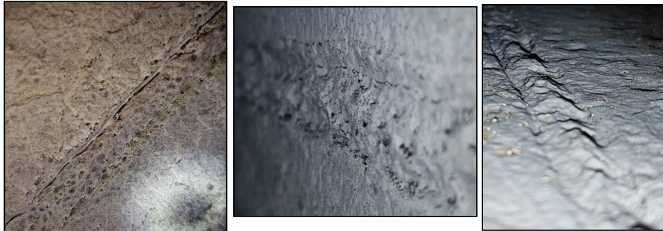
Figure 3-3: Longitudinal Seams in Penstock No.1 Section 16
