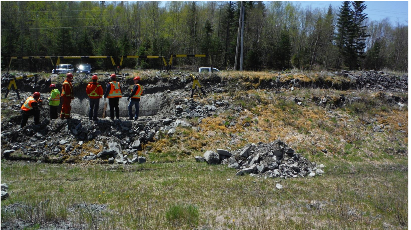
PHOTO 8 – LOOKING AT THE LEFT SIDE OF THE PENSTOCK IN AREA OF CRACK. NOTE SLUMPED BACKFILL
