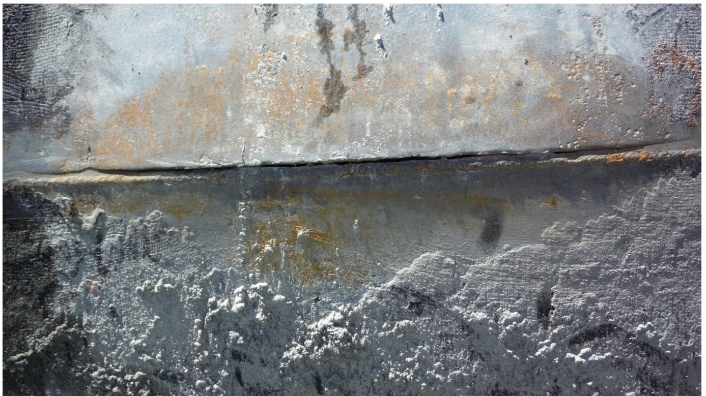
PHOTO 2 – CRACK IN PENSTOCK PLATE ALONG LONGITUDINAL WELD
