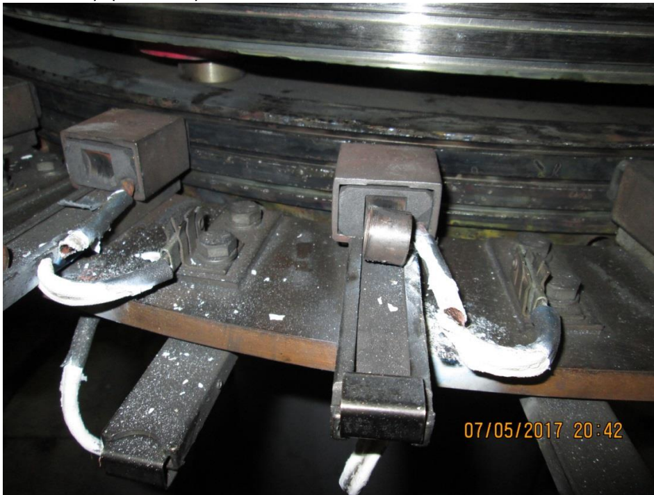
T5: There is arcing damage on one corner of the brush holder. The brush wear is at the threshold for replacement. The pigtail is melted off. The spring is broken. (Picture 7)
