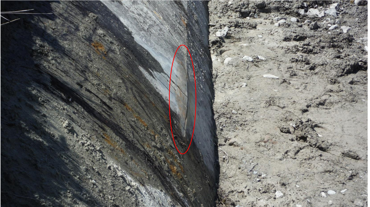
PHOTO 7 – LOOKING UPSTREAM FOR SIDE VIEW OF CRACK AND BULGE
