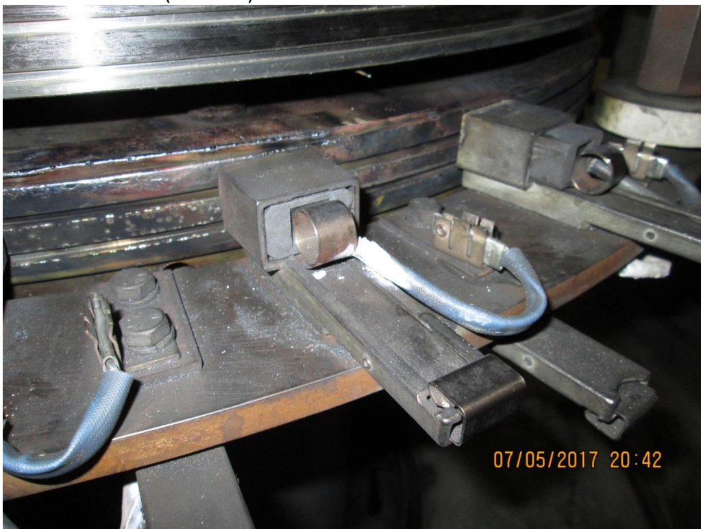
T3: The brush wear is at the threshold for replacement. The pigtail is melted off at the brush connection. (Picture 5)
