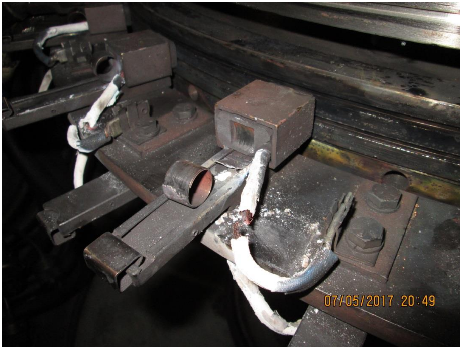
T9: The brush holder has pits / splatter on the top. The brush wear is at the threshold for replacement. The pigtail is melted off in the middle. There is full (poor) contact at the brush face. (Picture 12)
