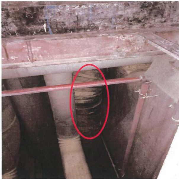
Exposed Pipe Insulation
