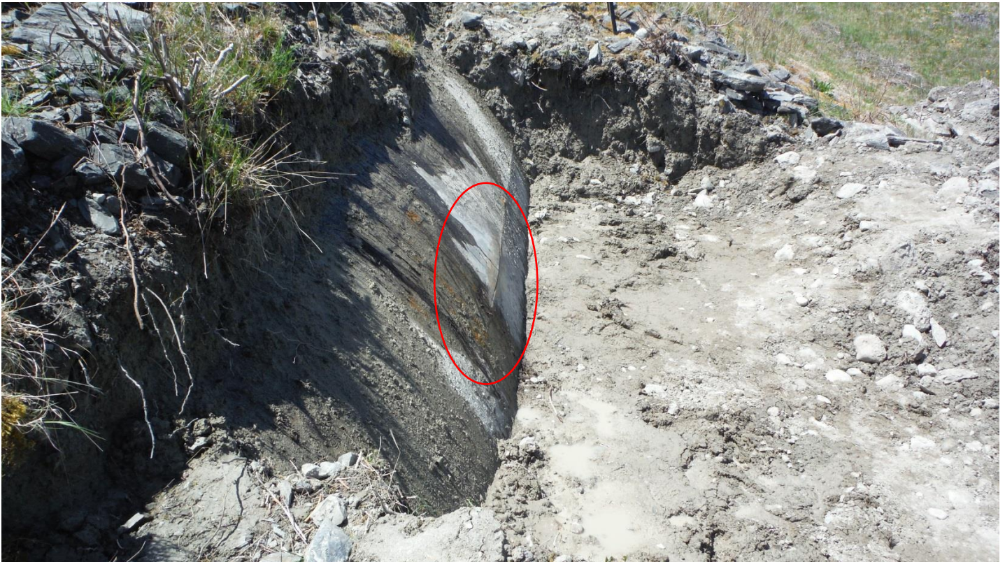
PHOTO 6 – LOOKING UPSTREAM ALONG CRACK LOCATION WITH BACKFILL REMOVED
