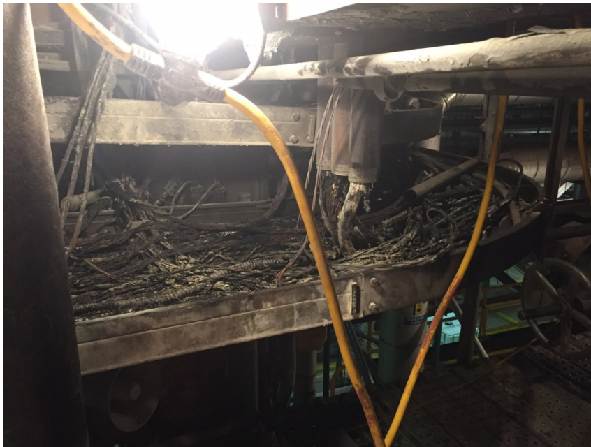
Figure 2 – Unit 2 Fire Damage (B)
