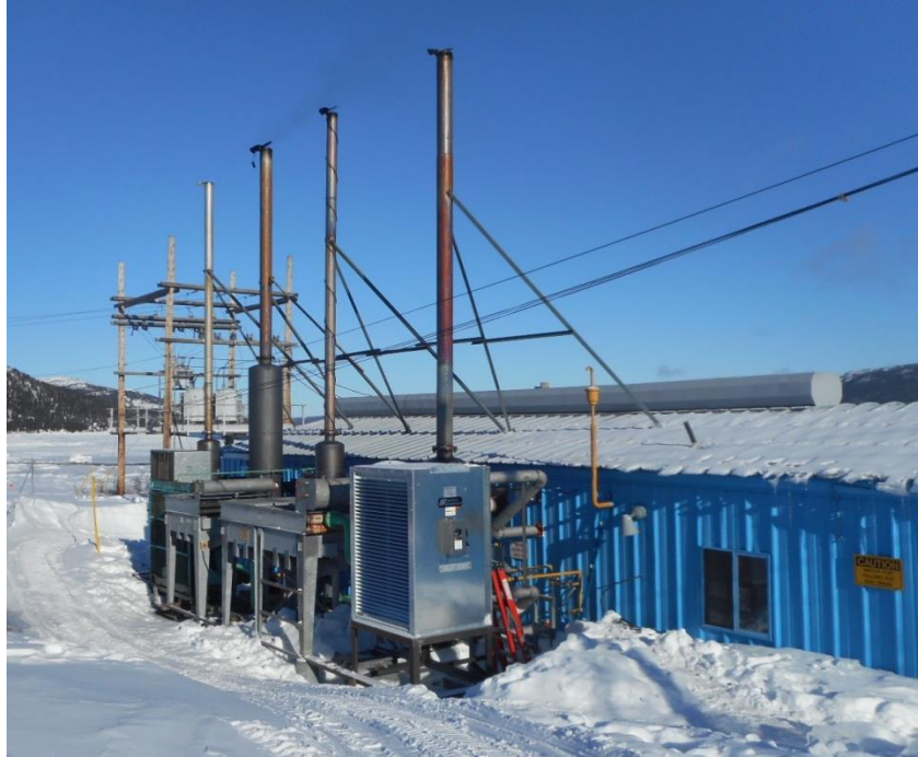
Photo 3: New Aftercooler Installed Outside the Rigolet Plant
