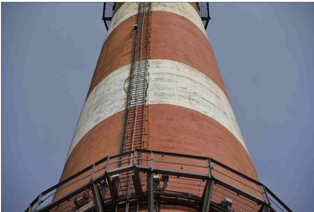
Photo 7: Stack No. 2 View from Powerhouse Roof Lower Section Above Lower Platform
