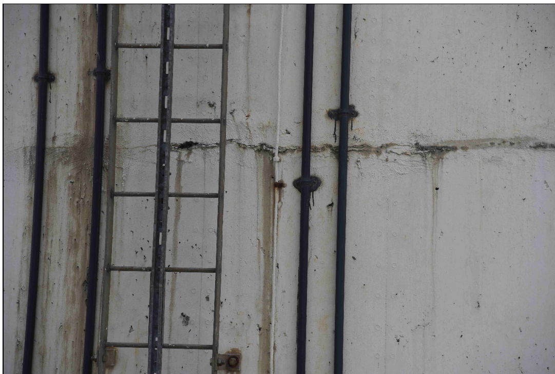
Photo 4: Stack No. 2 View from Powerhouse Roof Lower Section
