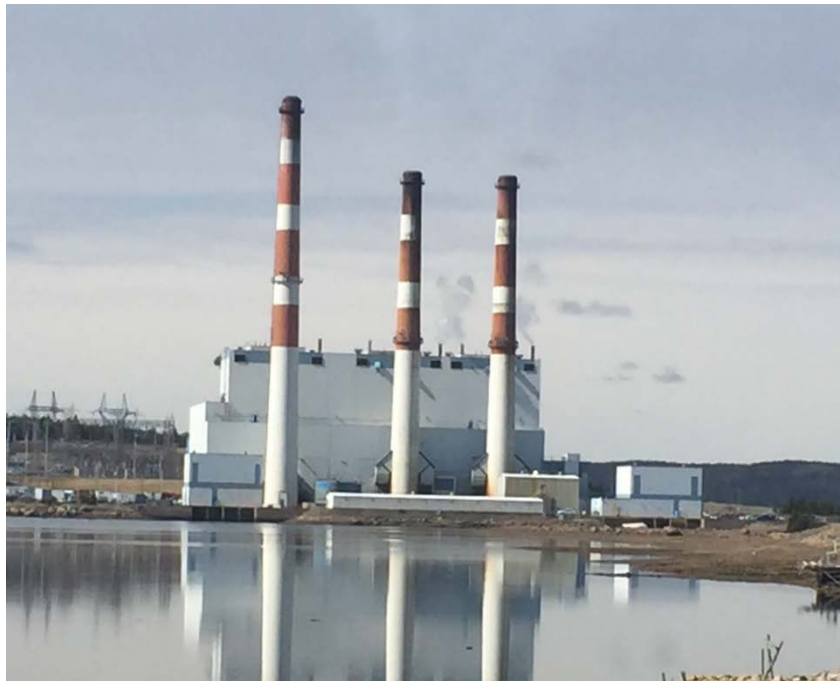
Figure 1: Holyrood Thermal Generating Station
