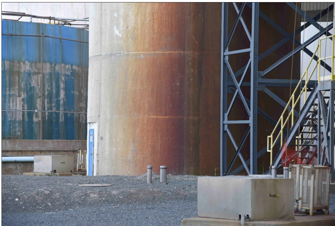
Photo 1: Stack No. 2 Lower Section
