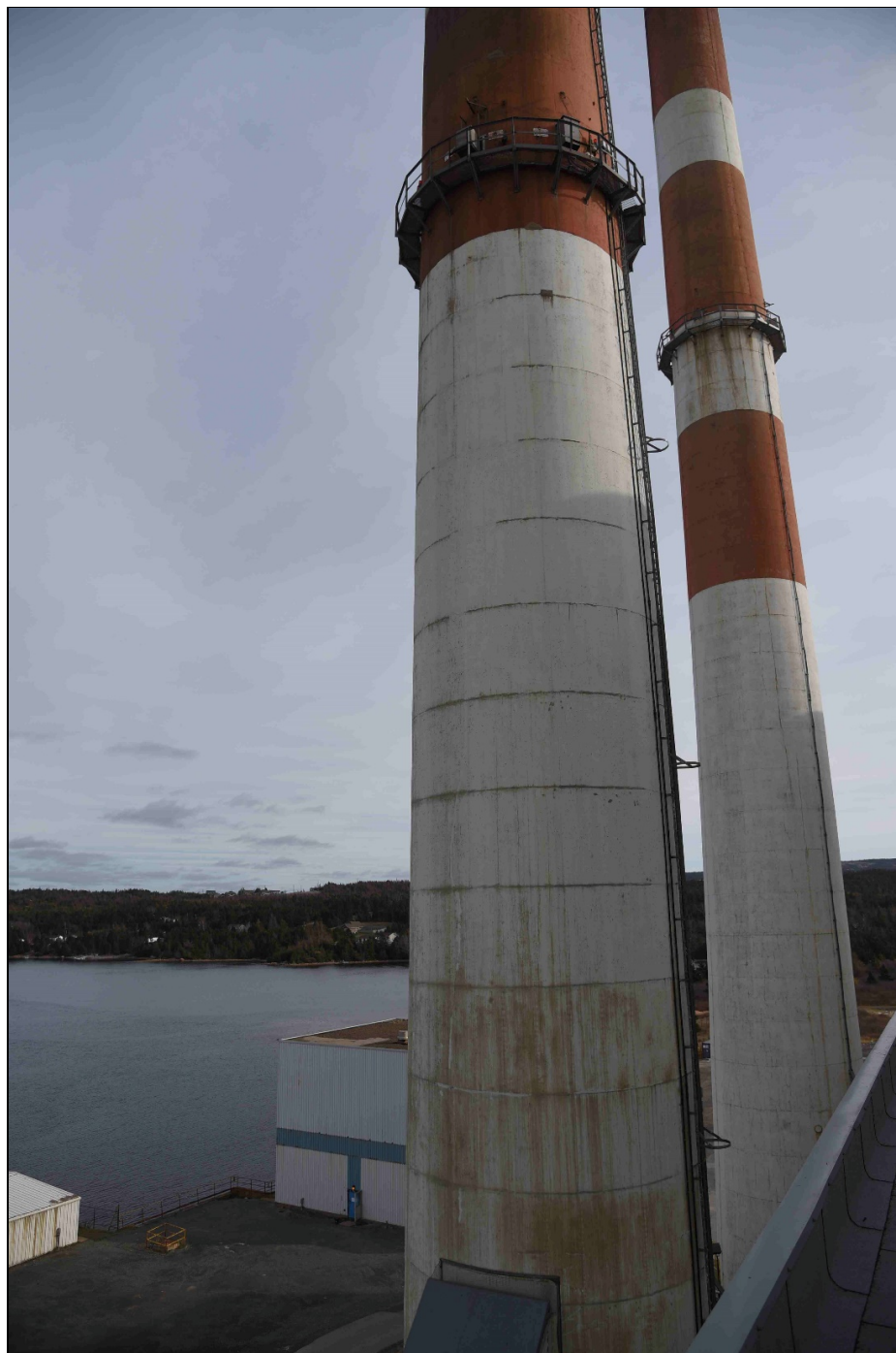
Photo 8: Stack No. 2 View from Powerhouse Roof Lower Elevation above Breaching Connection
