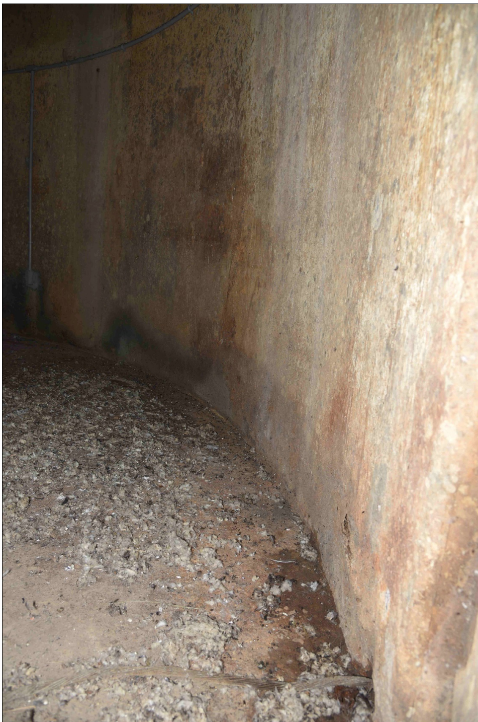
Photo 3: Tank No. 2 Interior View of Base Slab and Stack Interface
