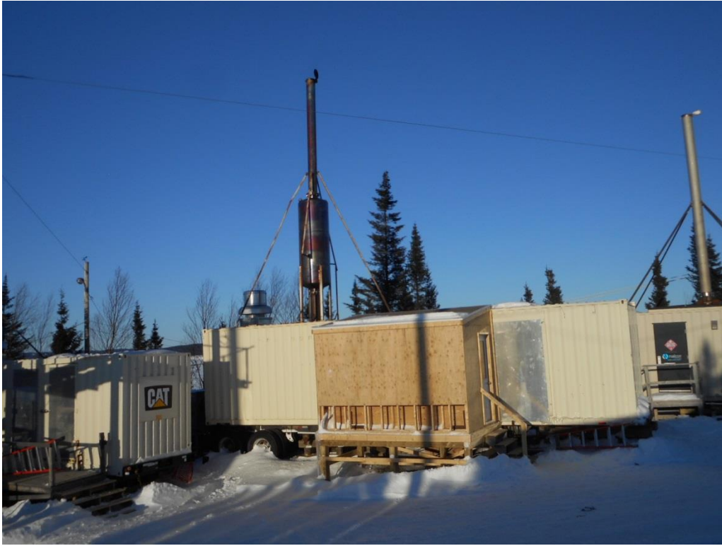
Photo 15: Overall Site – Units 2088, 2089 and 2102
