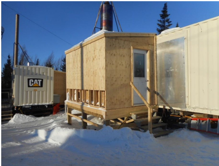
Photo 10: Unit 2089 Vestibule Complete
