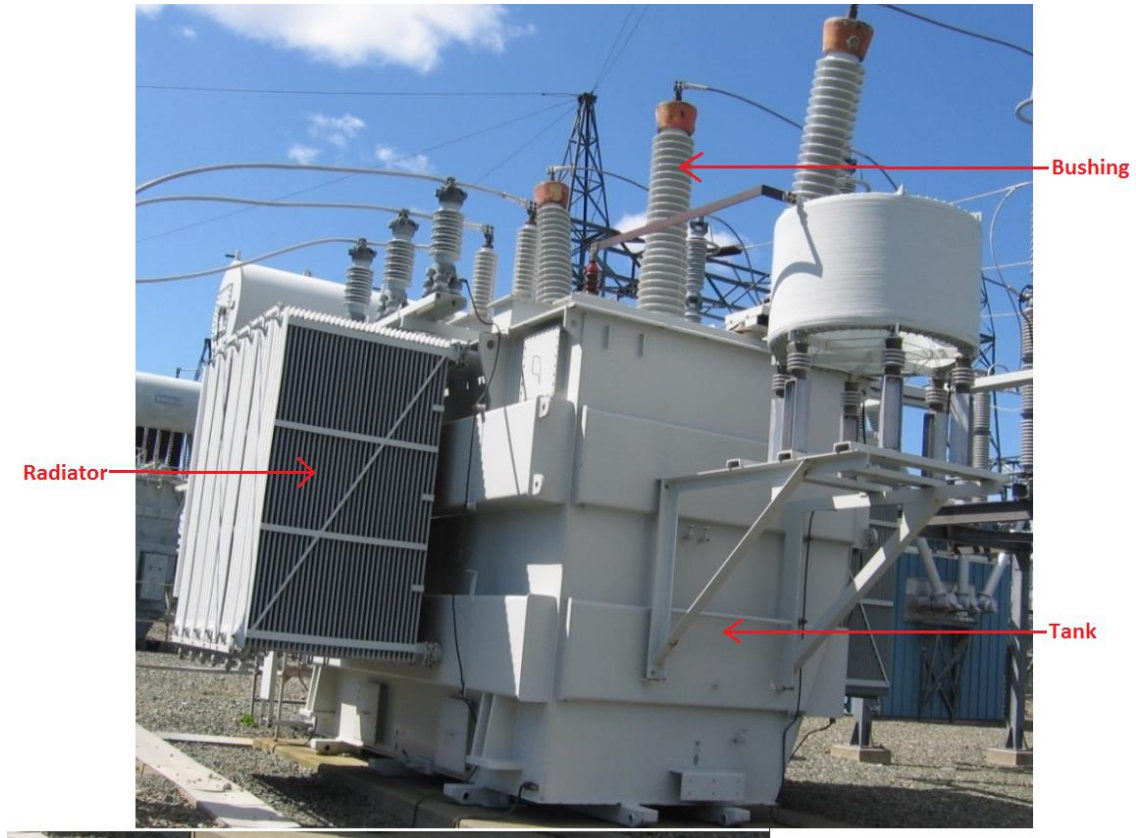
Figure 8: Power Transformer
