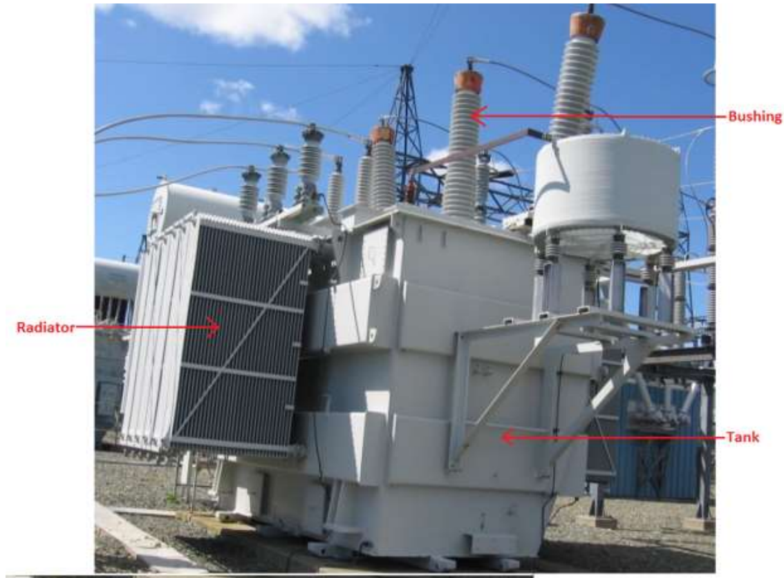
Figure 8: Power Transformer
