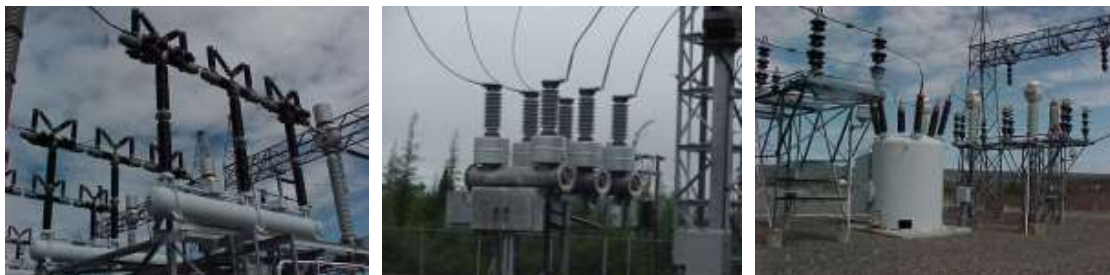
Figure 9: Air Blast Circuit Breakers (Left), SF 6 Circuit Breakers (Middle), and Oil Circuit Breakers (Right)
