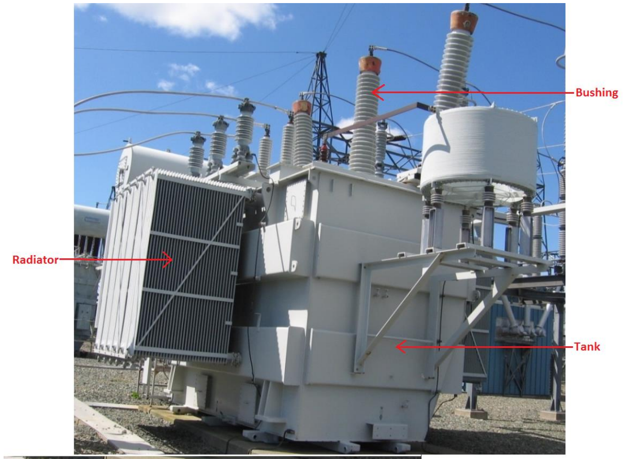
Figure 8: Power Transformer
