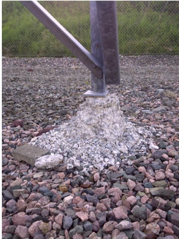
Figure 15: Structure L01L37-1 Western Avalon Terminal Station
