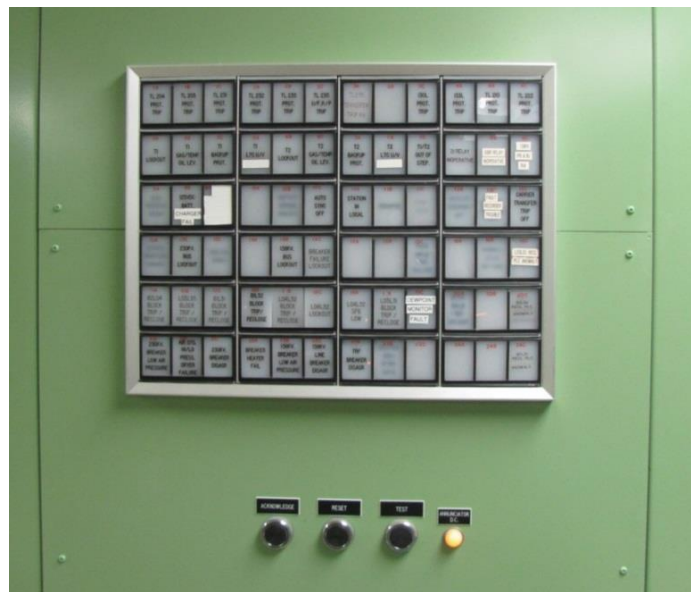
Figure 19: Annunciator Commonly Found in Hydro Terminal Stations
