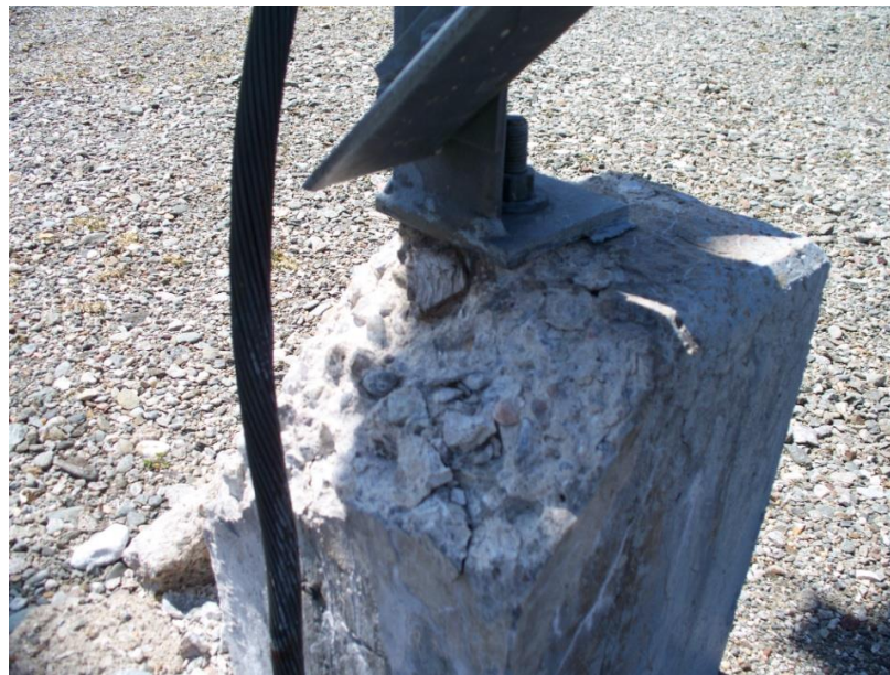
Figure 14: Structure B1T1 Bottom Brook Terminal Station
